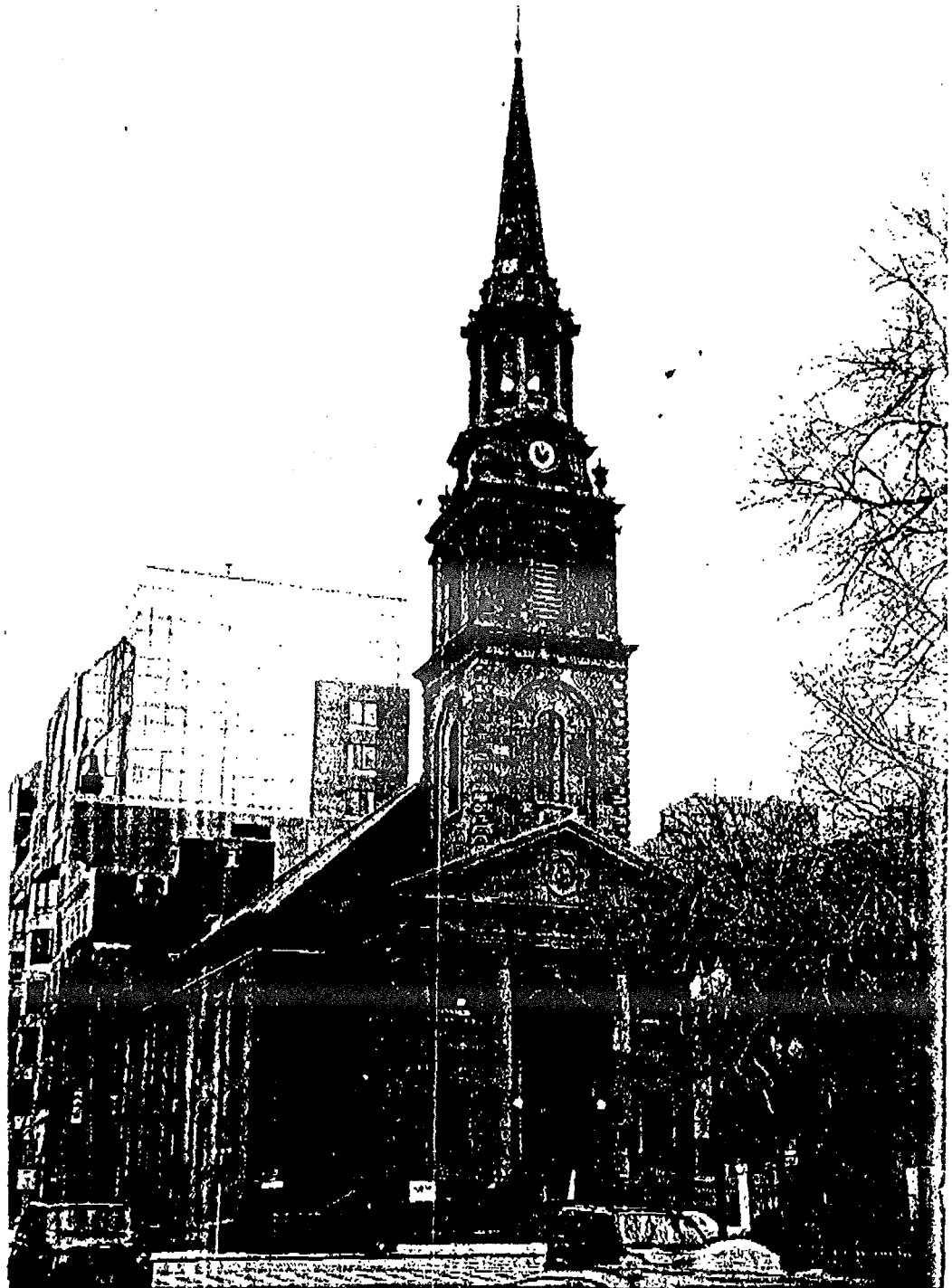
Arlington church steeple restoration by Northern Lights Painting Co., Inc.
