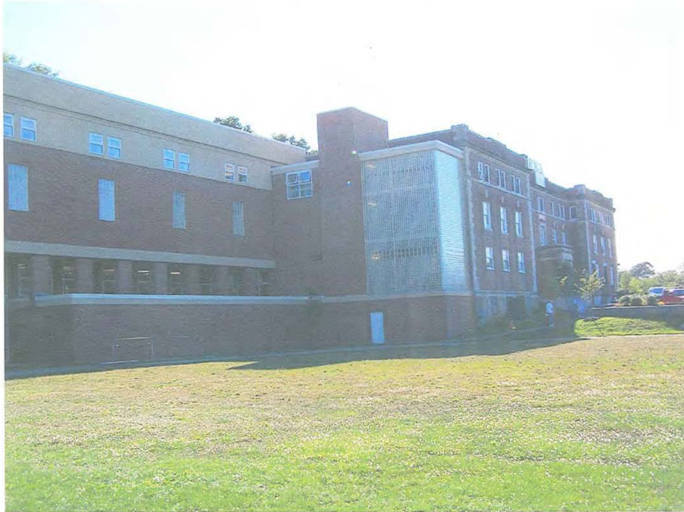
FRONT FAÇADE WITH NEW ADDITION
