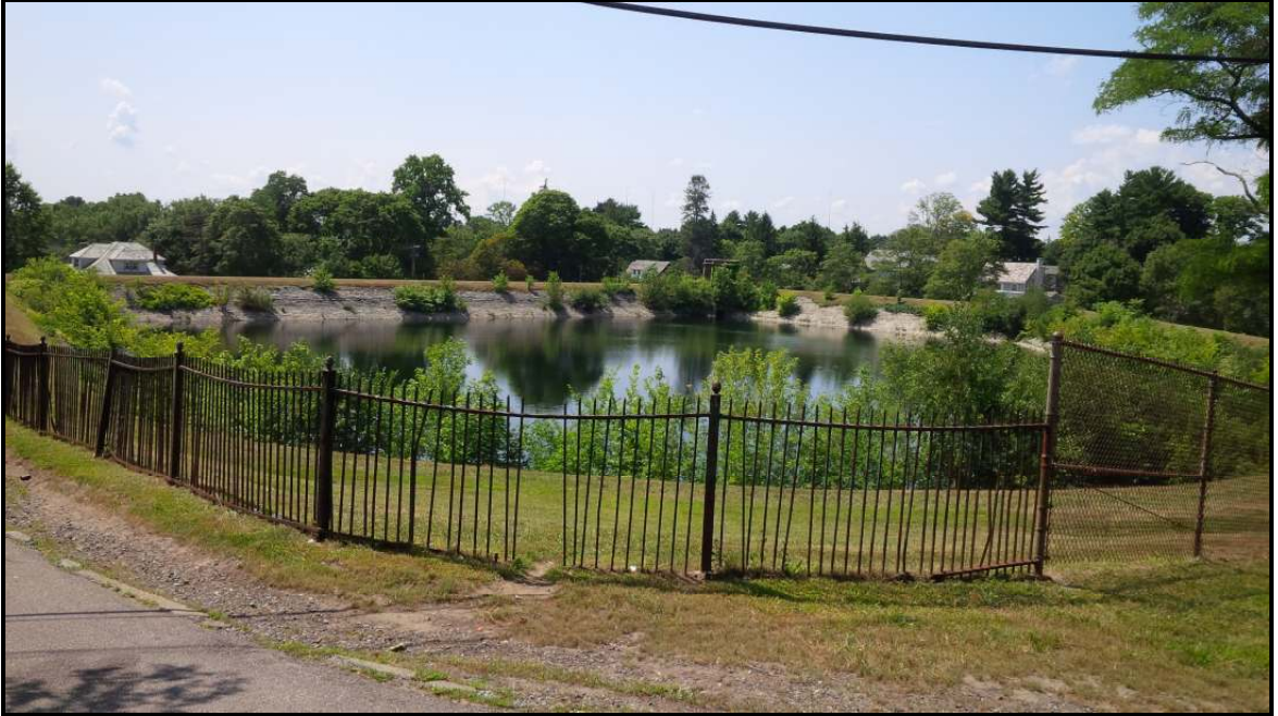
View of Reservoir, from Manet Road at Reservoir Drive
