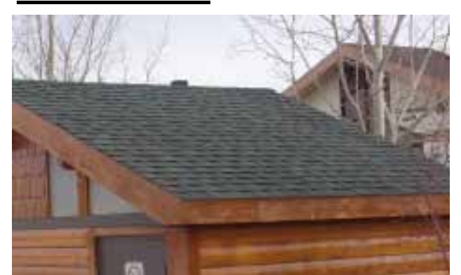
Asphalt Shingle Roof
