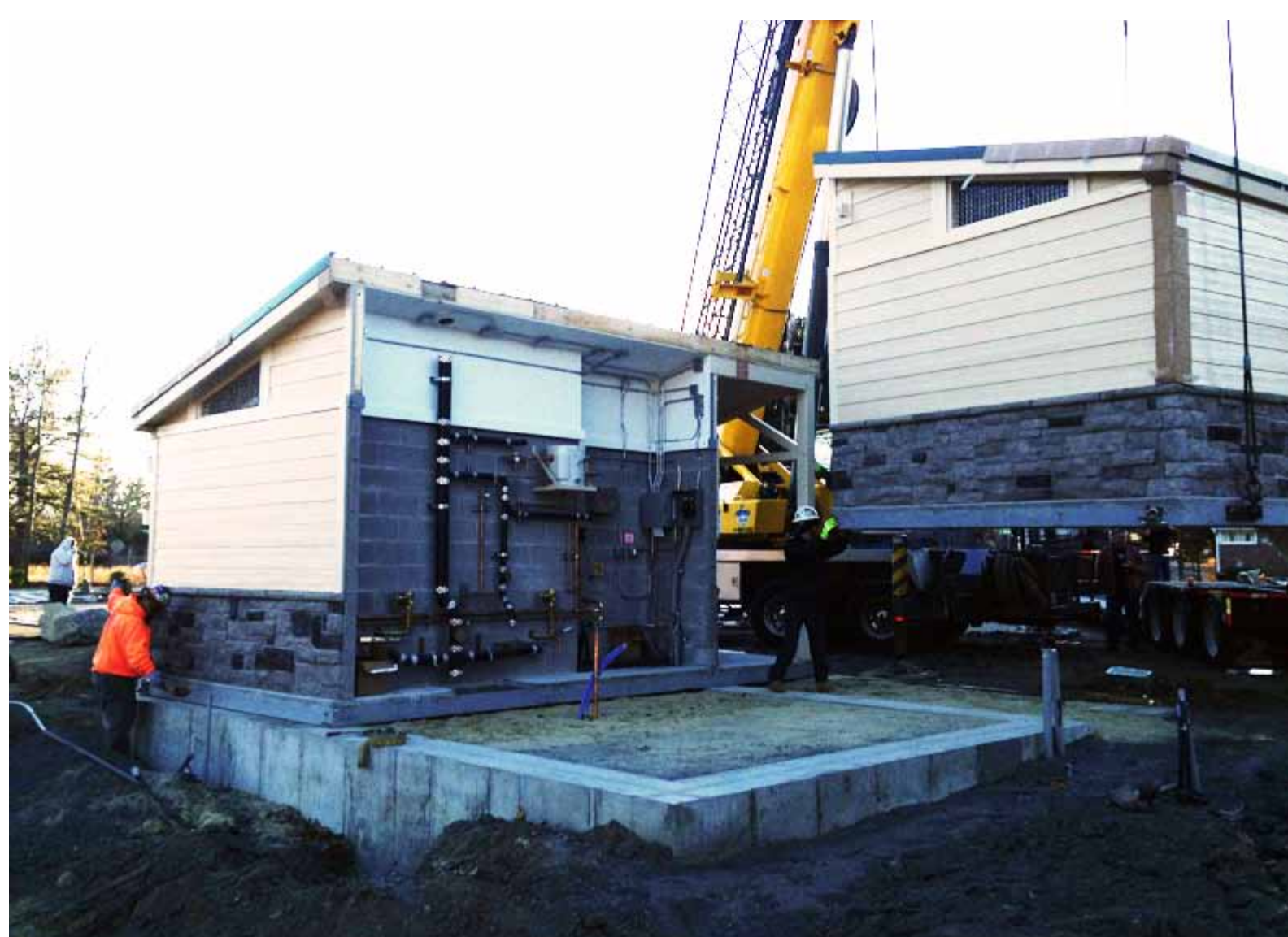
Example of building assembly. The modular building arrives on site fully plumbed and wired. It is then craned over the foundation and pad, with utilities stubbed up by the site contractor. Once the building is in place, final connections are made within the utility chase.
