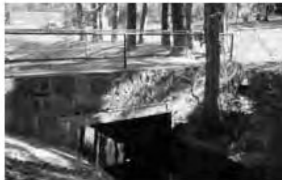
Bridge over Hammond Brook, 2005
