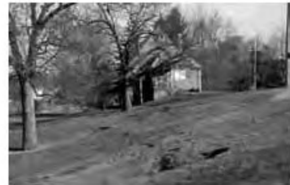
Erosion near Recreation Center, 2005
