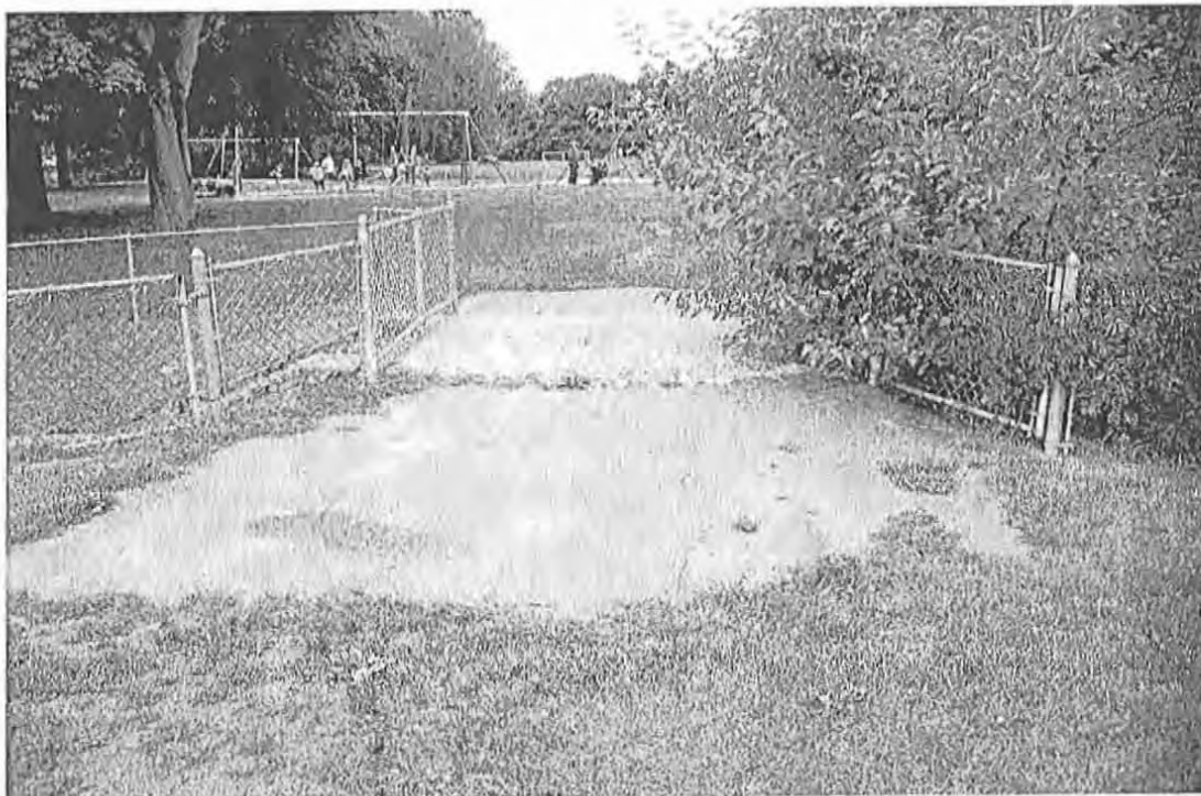
EXISTING FOOTBRIDGE OVER BROOK LOOKING WEST
