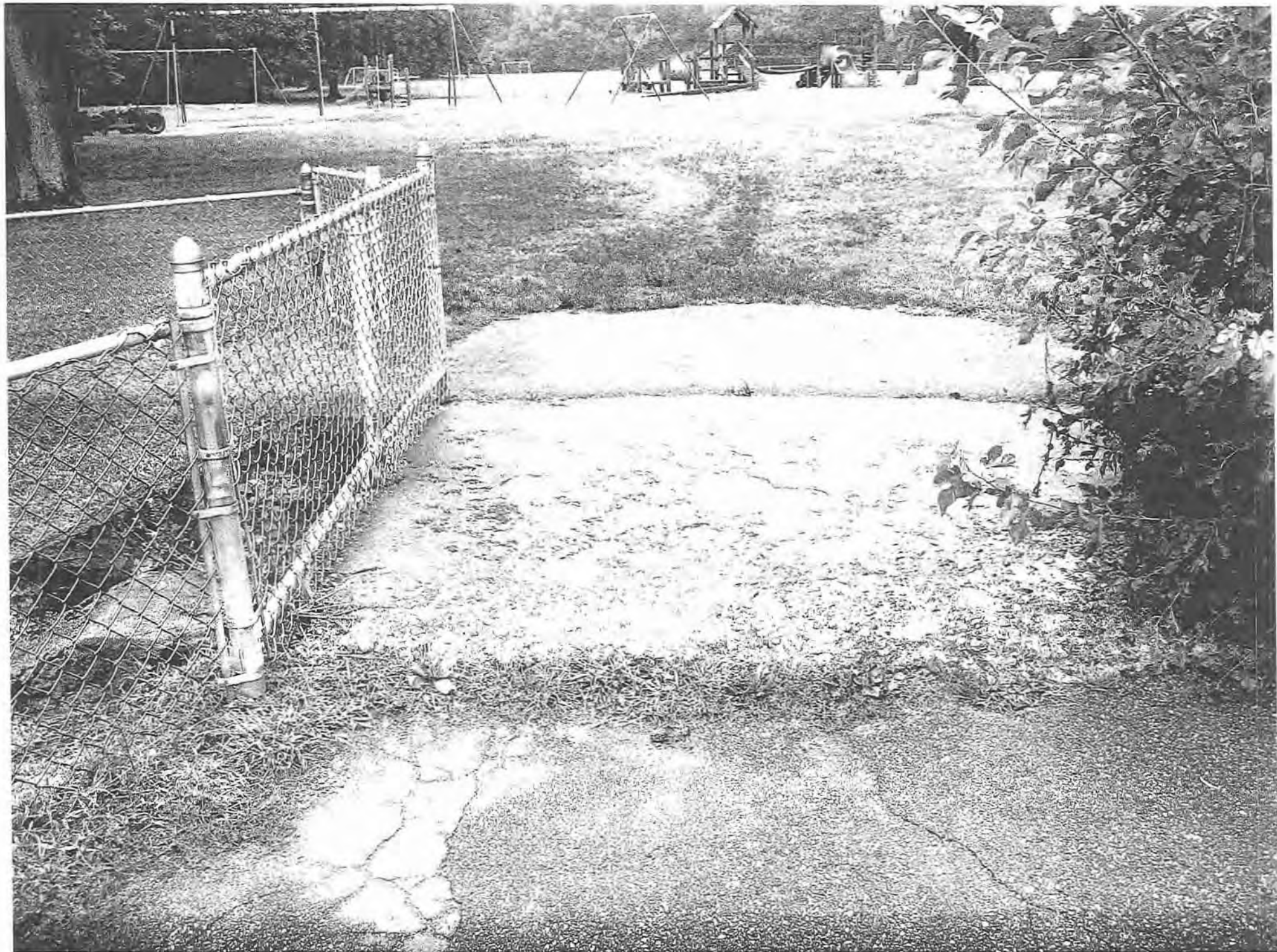
BRIDGE OVER BROOK TO PLAY AREA
