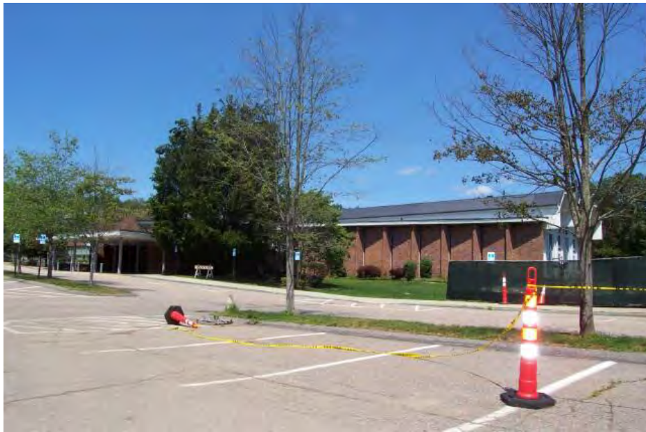
View Looking NW at the Subject Building.
