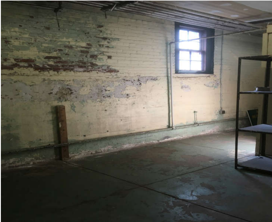
Photograph No. INT-06
