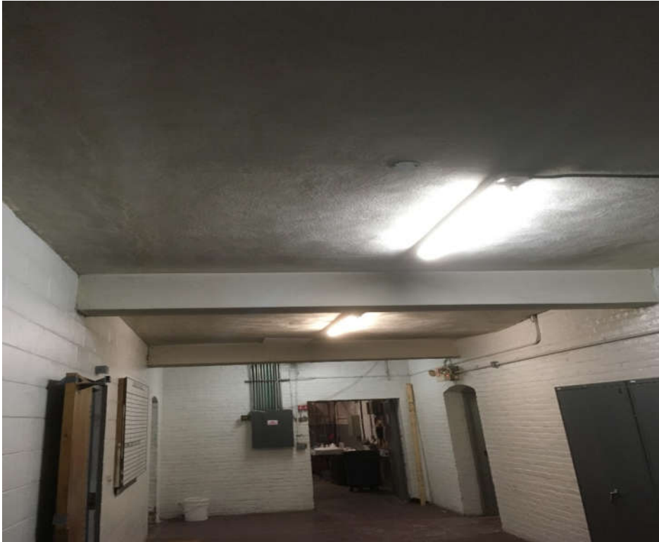
Photograph No. INT-07
