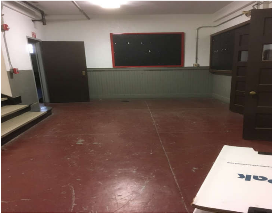
Photograph No. INT-09
