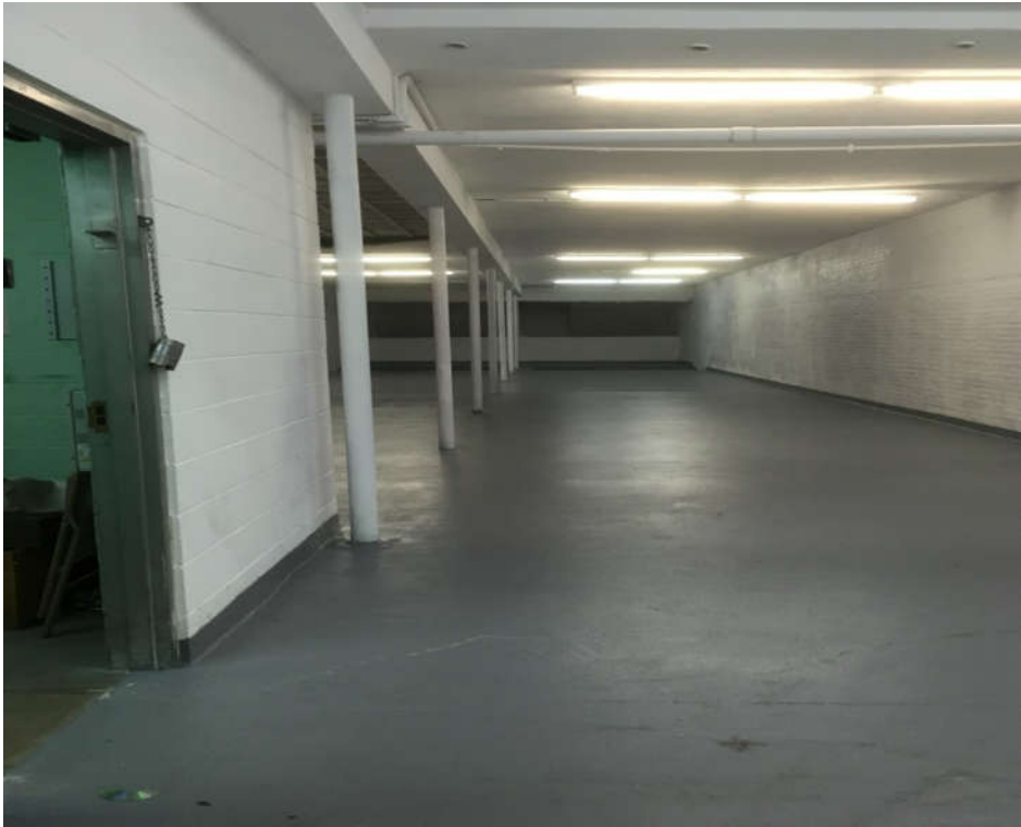
Photograph No. INT-05
