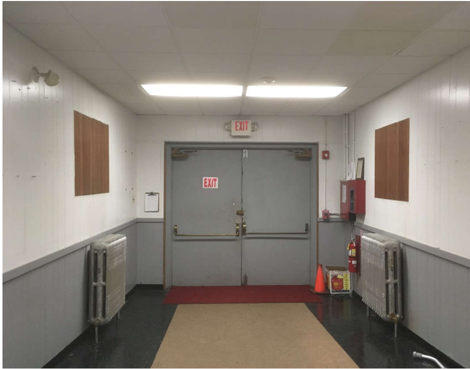
Photograph No. INT-02
