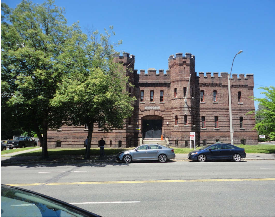
Photograph No. EXT-01 Building south entrance
