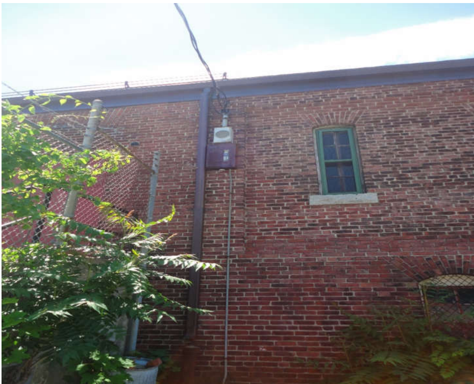
Photograph No. EXT-02 Partial east elevation with overhead electric service
