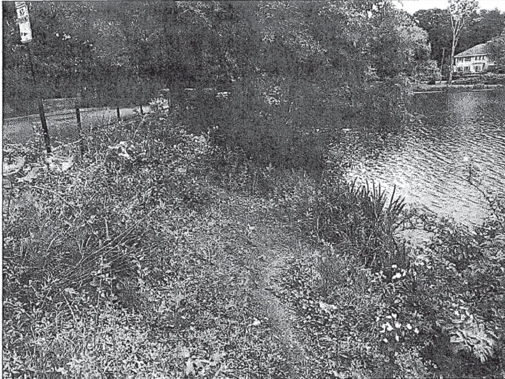
Photo No. 1: Upstream slope right of the low level outlet.
