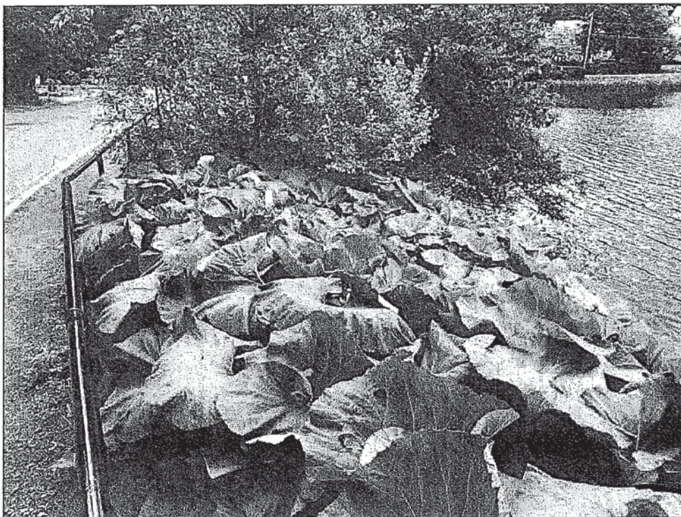
Photo No. 2: Upstream slope right of the spillway.
