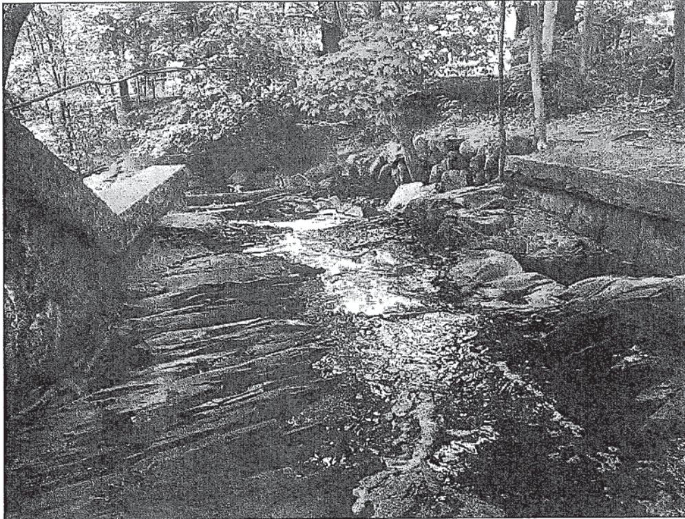
Photo No. 9: Downstream channel at the spillway.
