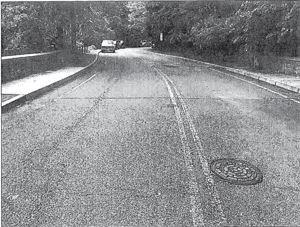
Photo No. 3: Crest from near the right abutment looking left.
