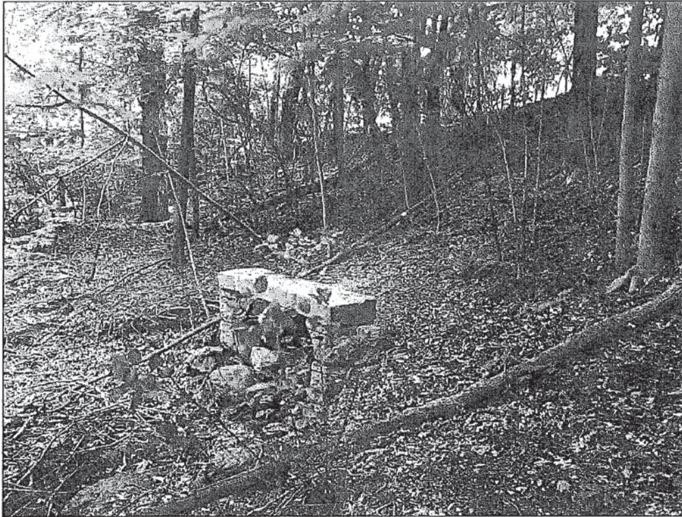
Photo No. 5: Downstream slope from near the left abutment.
