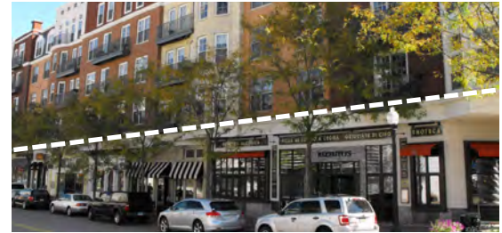
Ground floor storefront continuity
