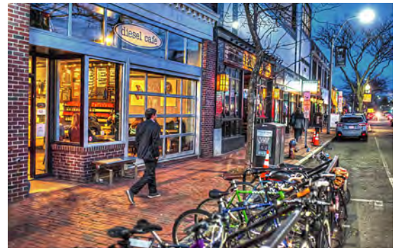
Ground floor transparency creates a vibrant street
