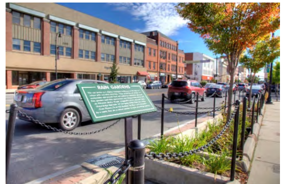
Bioretention Planters North Street, Pittsfield
