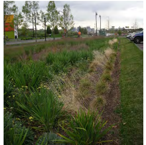
Bioretention Basin Assembly Row, Somerville
