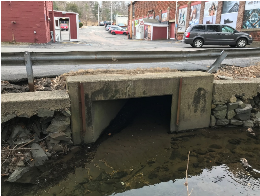
Existing 4' x 5' box culvert outlet at Cheesecake Brook
