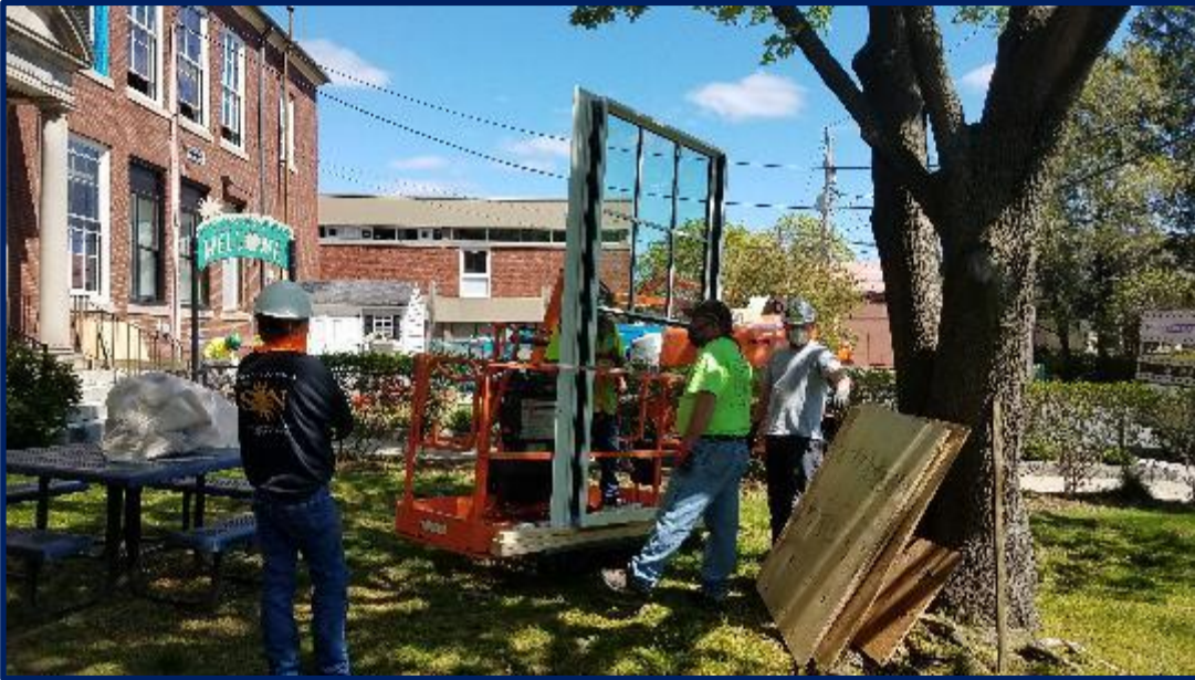
Replaced 350+ windows and doors, boiler and temp control systems
