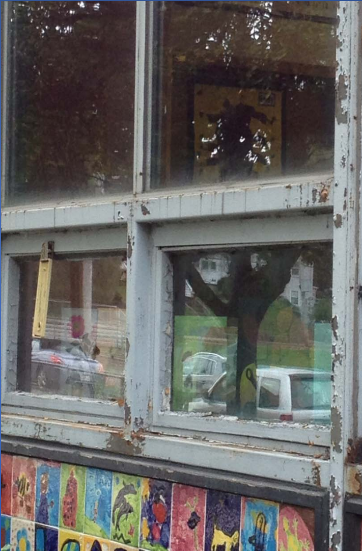
Cabot – Window and Door Deterioration
