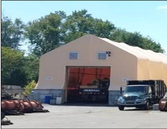
Constructed in 2014, this facility is 3,570 square feet and is used for equipment and vehicle storage. The building is a fabric membrane, stretched over a steel structure, with a v-block concrete foundation.
