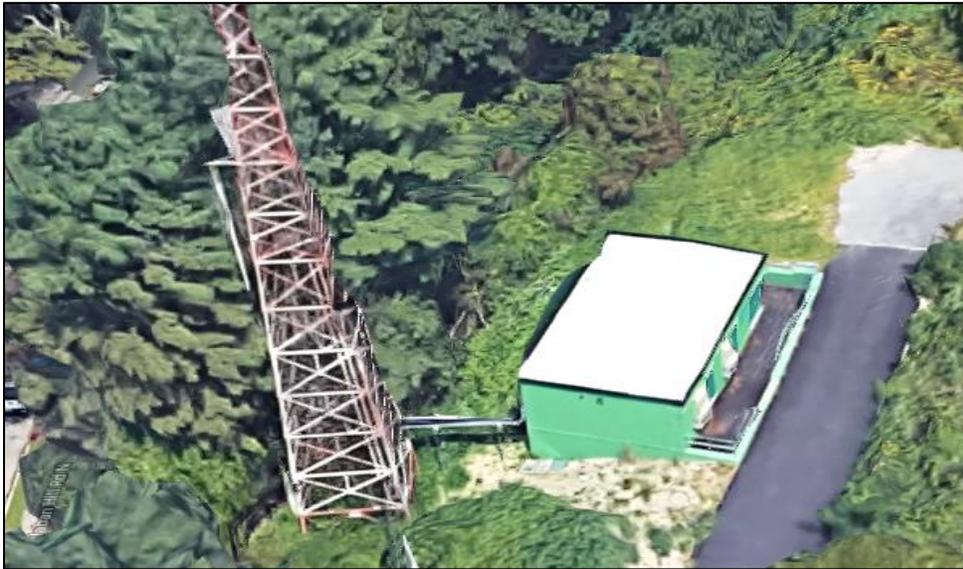
Built in 2016, this 836 square foot prefab concrete building houses communications equipment.
