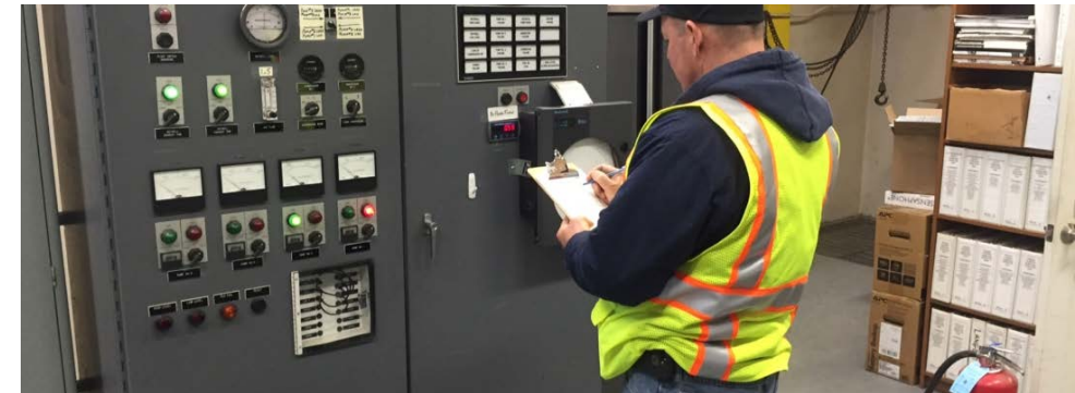
Pump Station Assessment Upgrades Project
