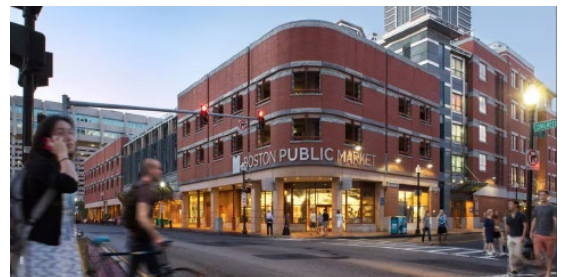
Ground floor commercial liner in parking structure
