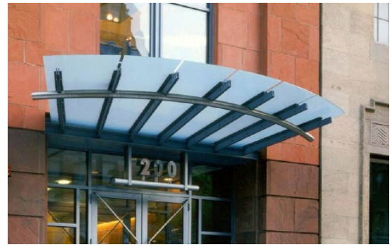
Added architectural detail at building entries
