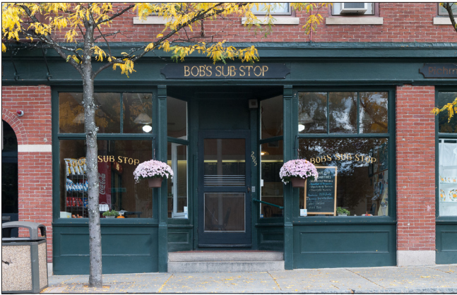
This historic storefront in Newton Upper Falls is an important element of the streetscape. Note the location of the commercial signage, applied to both the storefront glass and the storefront cornice above the entry door.
