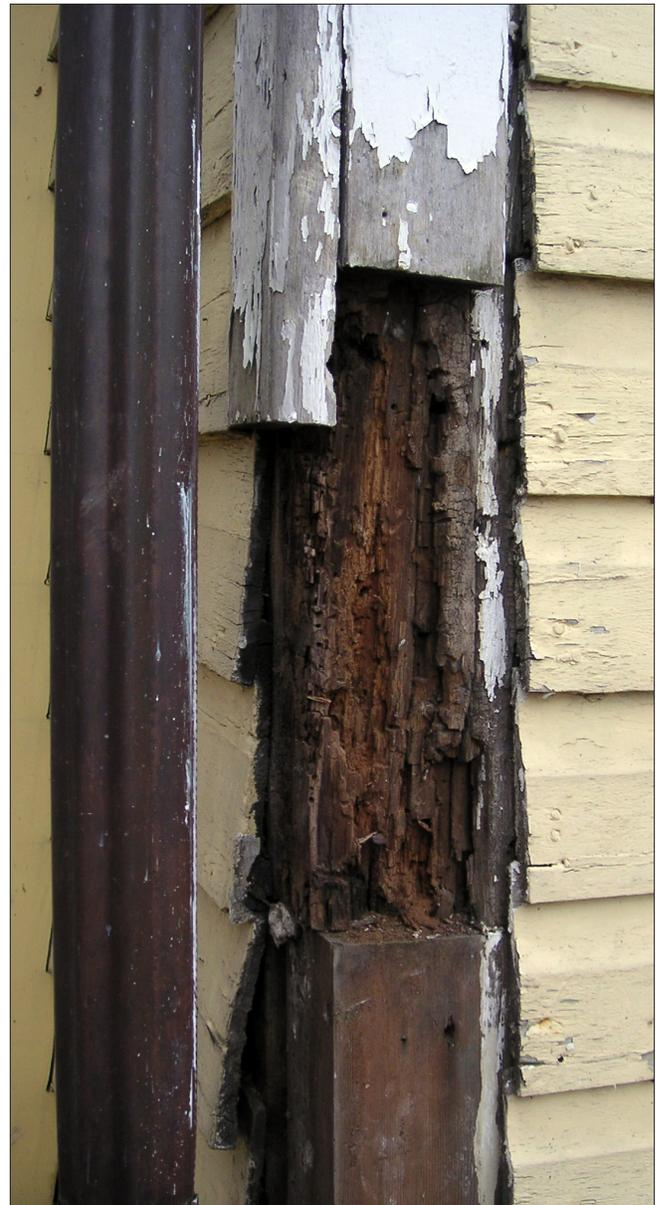
*The vertical wood corner boards were removed adjacent to the downspout exposing the structural wood post. Additional exploration revealed that there was significant rot of the post that extended deep into the thickness of the wood, compromising the structural capacity. It is likely that a persistent leak at the juncture of the roof gutter and downspout made the situation much worse.*
