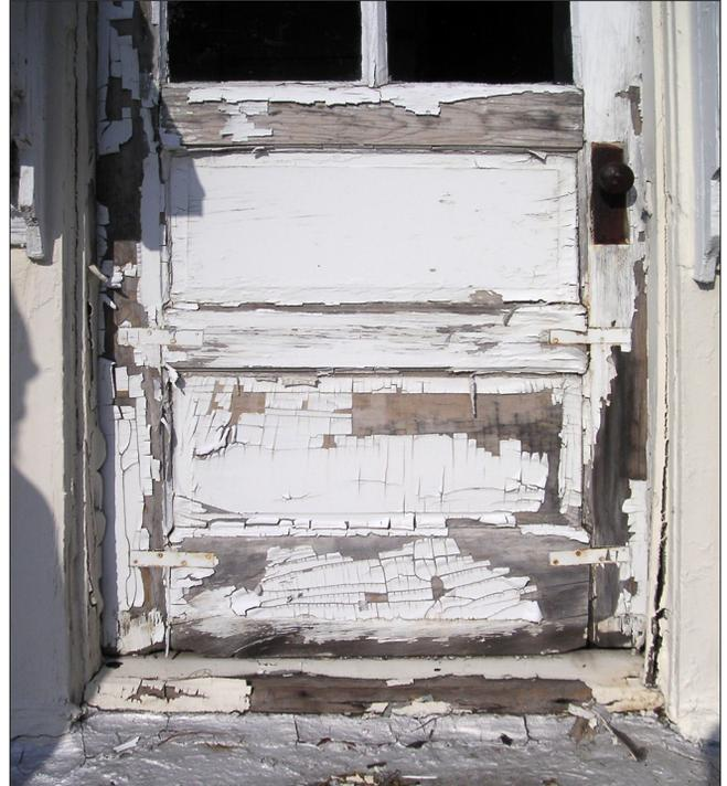
*The paint on this door has alligatored, and severe cracking is visible. Removal of paint down to bare wood and proper door repair are recommended prior to repainting.*
