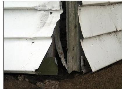
*Aluminum and vinyl siding were sometimes installed to conceal an underlying problem. In some cases, removal might be necessary to repair a deteriorated condition.*
