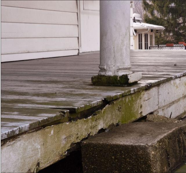
*Porches, steps and other areas where the woodwork is laid horizontally or located close to the ground are often first to deteriorate. Ongoing exposure to moisture can lead to rot of the column bases, porch deck and apron.*
