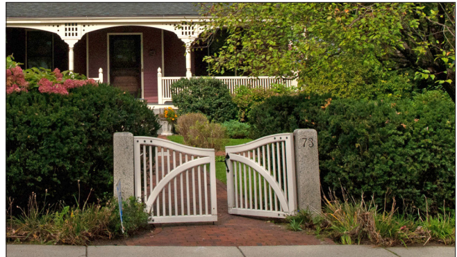
The wood gate is mounted on stone piers. The arched form complements the bays of the front porch.
