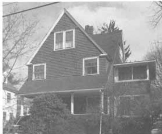
Figure 26. Shingle, 36 Oxford Road, built 1894
