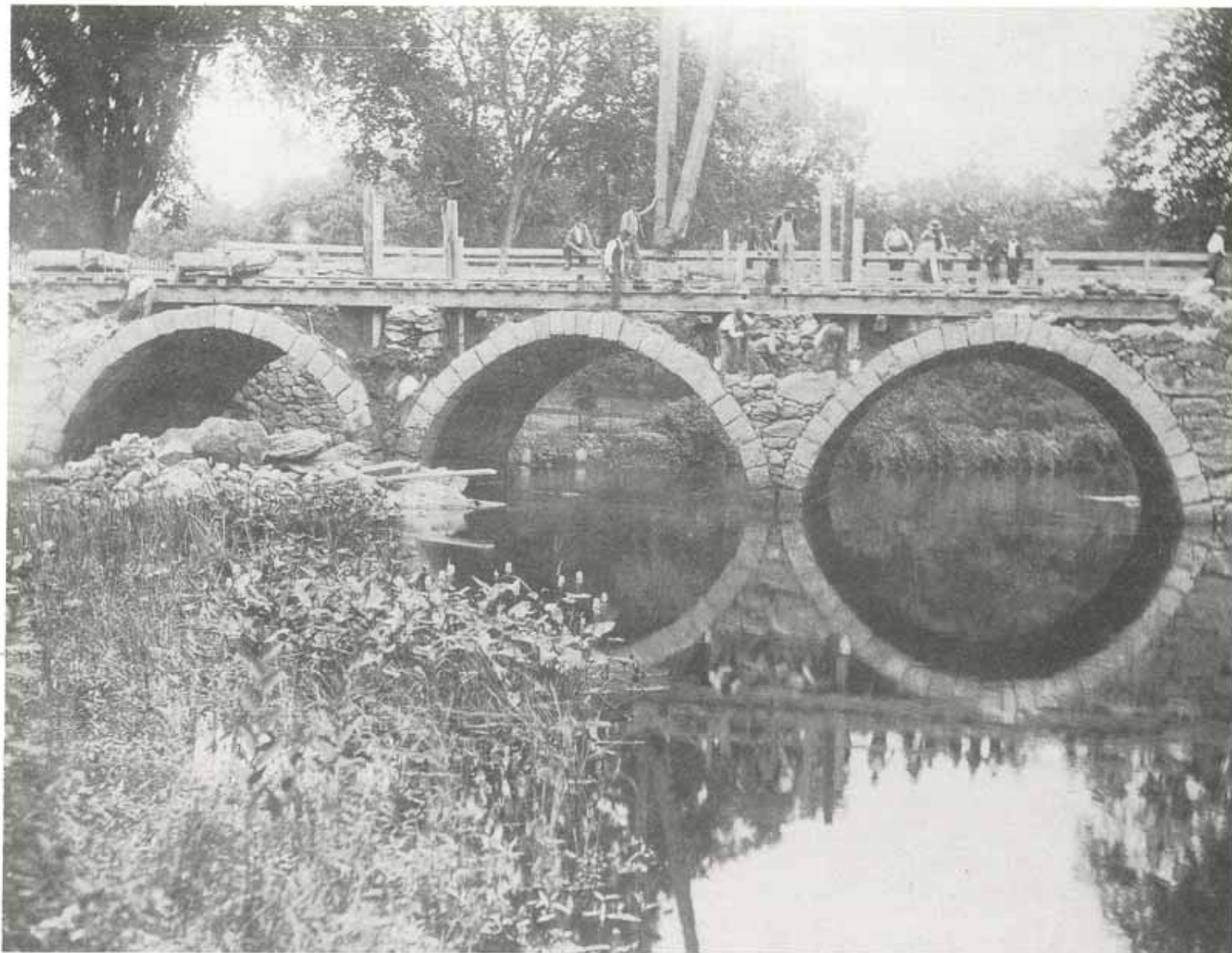
Cook's Bridge (Elliot Street-Central Avenue), Newton Upper Falls. Rewidening to accommodate streetcars to Needham, 1906
