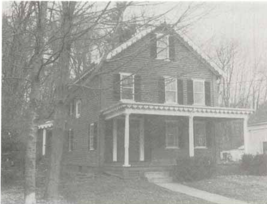
Figure 21. Lower Falls: 656 Grove Street, 1845
