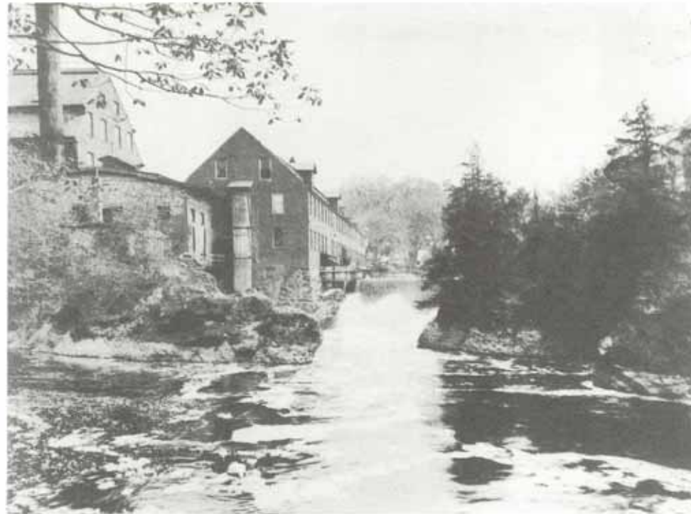
Development at Upper Dam, c. 1880 (Elliot Mills)
