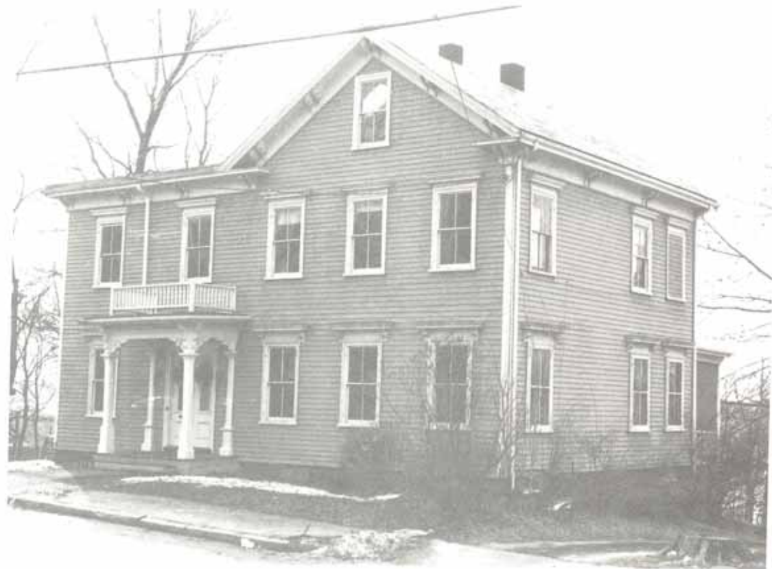
Figure 23. Upper Falls: 68 High Street, 1876
