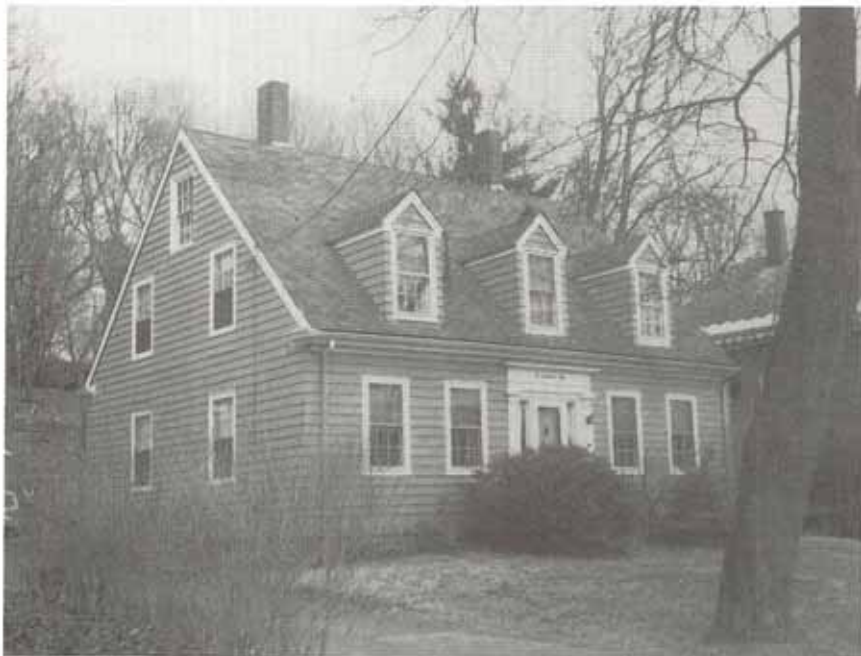
Figure 13. Lower Falls: 650 Grove Street, 1837-1838
