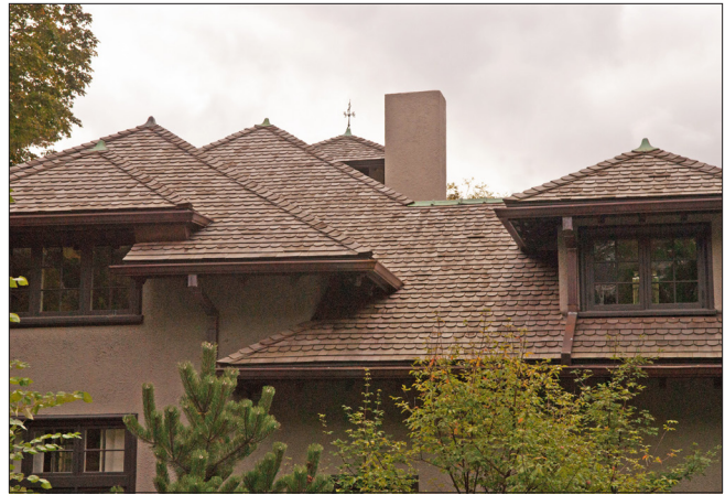
Wood shingle roofs can be applied in a variety of decorative patterns and configurations. This example includes alternating rows of scalloped and square-butt shingles.
