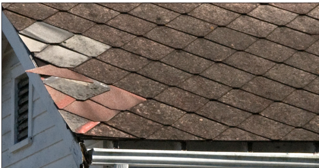
Asbestos roofing shingles came in various shapes, with diamond-shaped being the most common. This asbestos roof has some non-asbestos replacement shingles of similar size and shape as the existing roofing.
