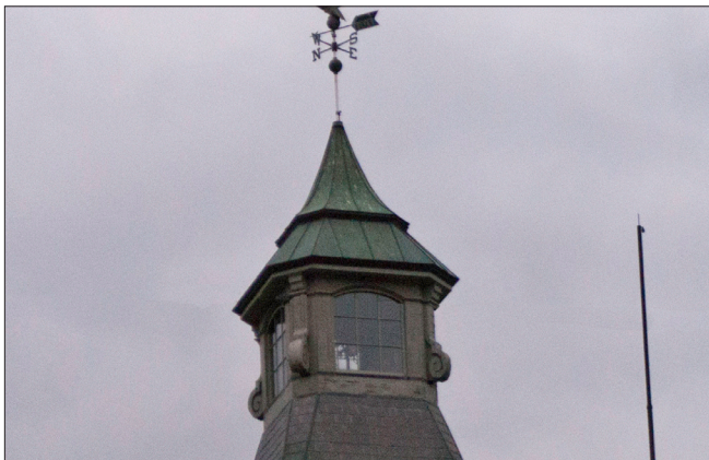
Metal standing-seam roofs were popularized in the mid-19th century. Decorative or unusually shaped roof elements, such as this cupola, were often covered with metal roofing.
