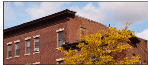
Flat roofs with parapets are frequently found on commercial or institutional buildings
