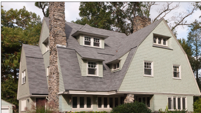
Dormers can be a significant character-defining element of a historic house. Gambrel roofs typically have dormers to increase habitable space at upper floors.
