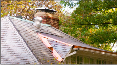
Flashing is commonly found at chimneys, dormers and intersections of roof forms.
