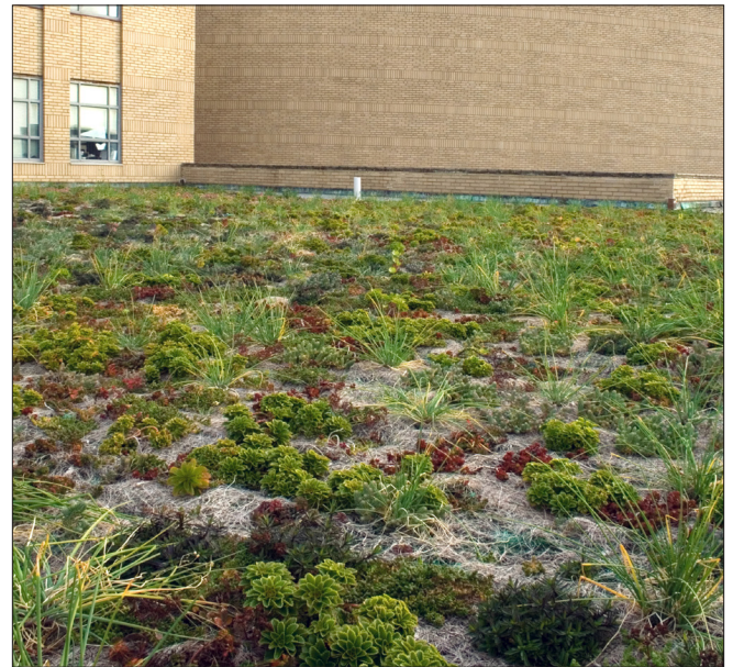
Green roofs are becoming increasingly common in new construction, providing both an insulating layer of soil and reduced stormwater runoff. They may be an energy-upgrade option for historic structures with flat roofs and sufficient structural capacity.
