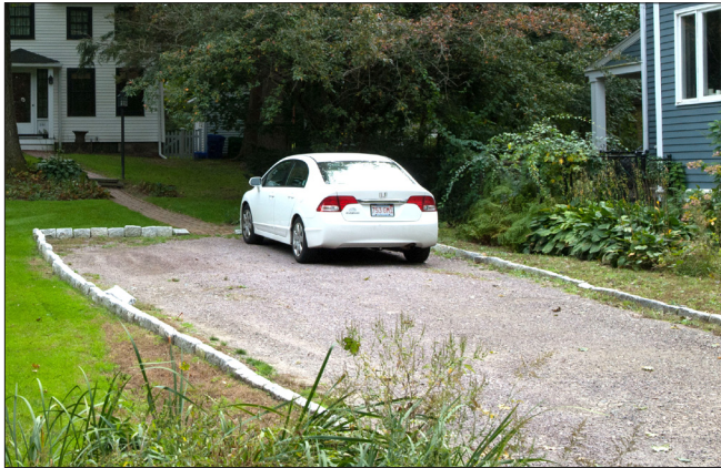
Sustainable site features - such as this permeable parking surface in Auburndale - can contribute to the overall sustainability of a property.
