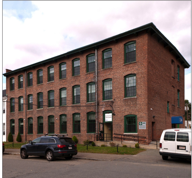
Many historic structures, such as this former industrial building in Newton Upper Falls, include numerous large windows that allow natural light and ventilation for the interior.
