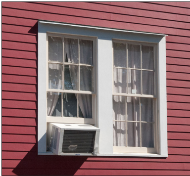
Installing window air-conditioning units in historic buildings is not encouraged, due to their appearance, likelihood of damaging windows and frames, and low efficiency.
