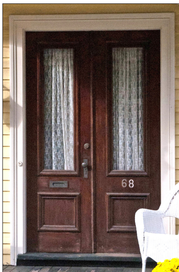
Paired wood doors, which often include glass lights, are typical of Victorian period buildings.
