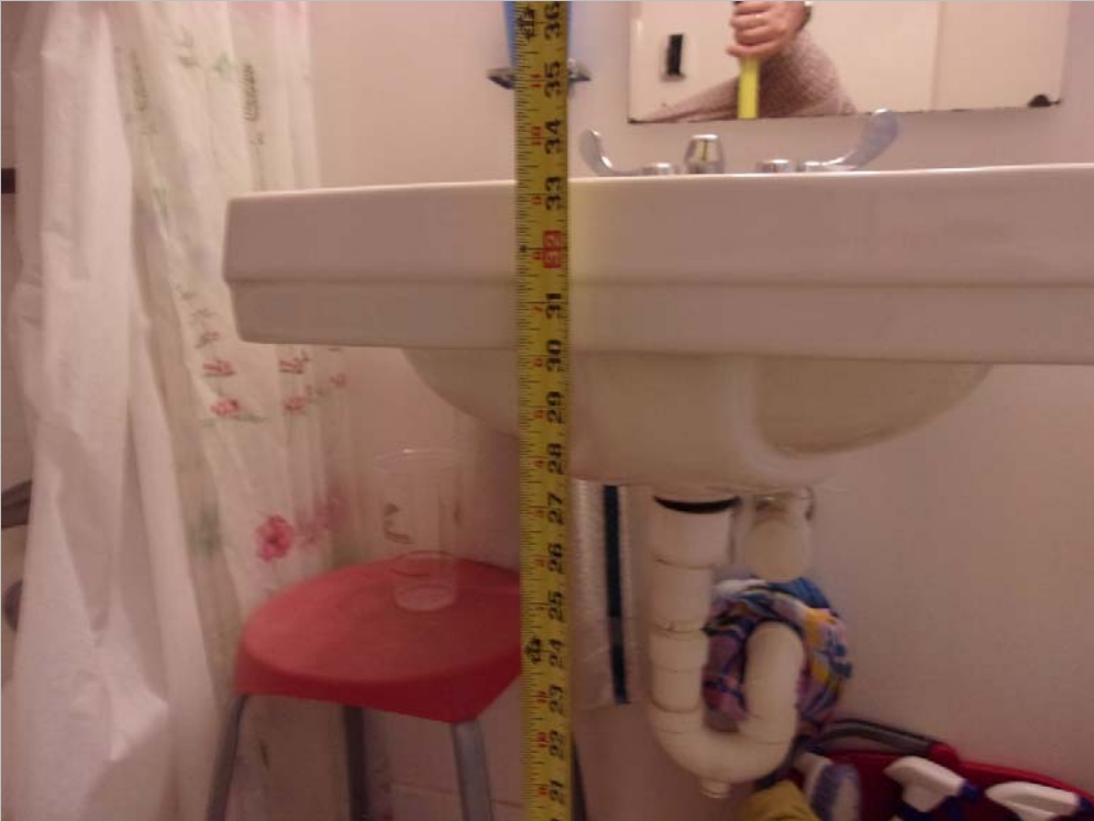
Handicap dwelling unit bathroom sink with scald and abrasion protection and levered hardware
