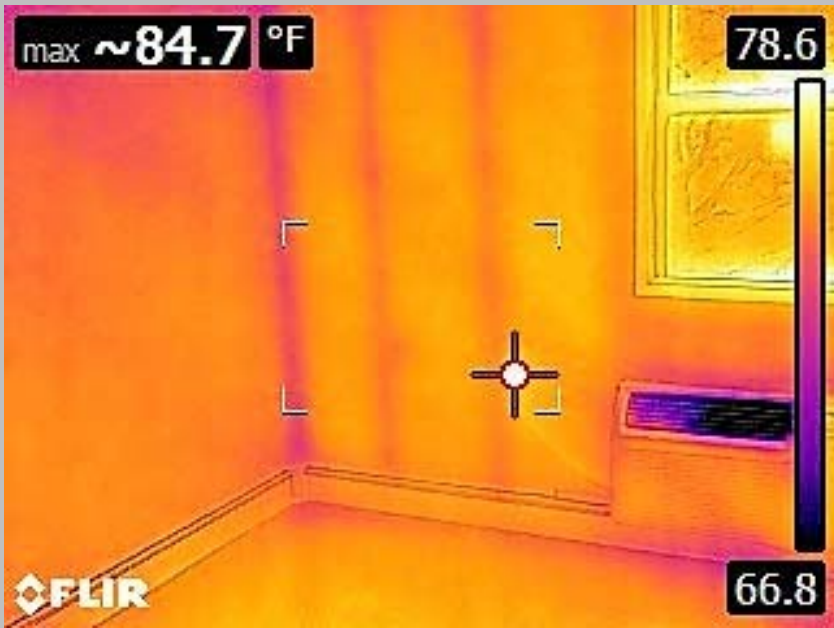
Thermal Image of Dwelling Unit Exterior Wall Without any Moisture Detected
