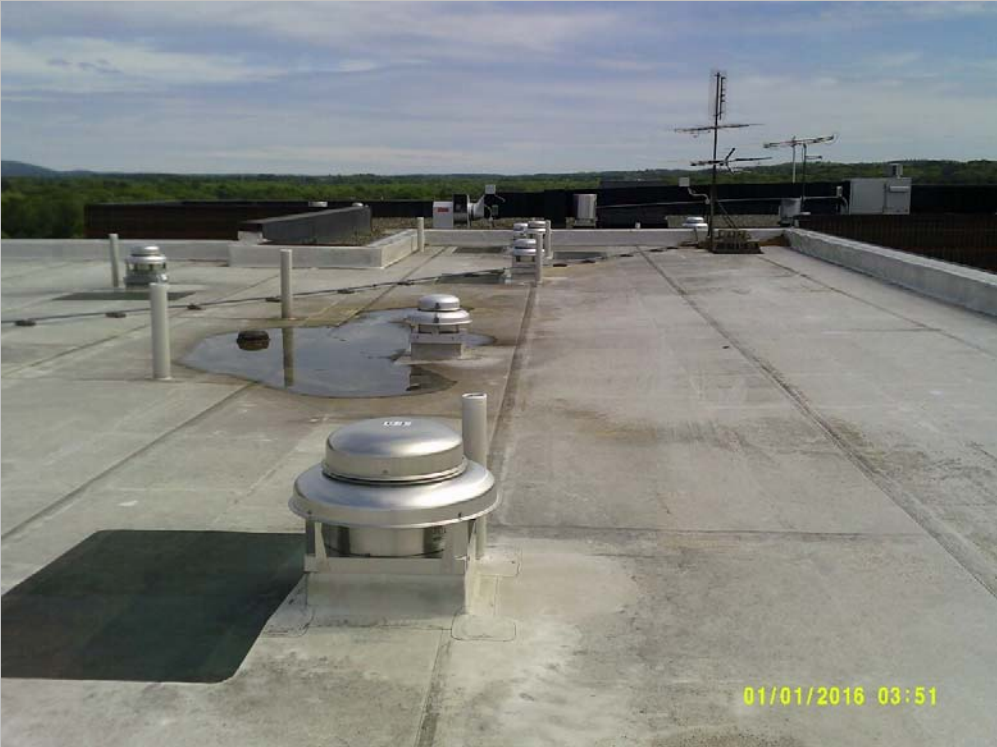
Coleman House I roof
