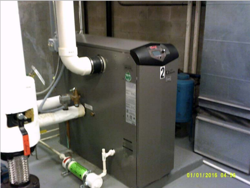
Gas-fired boiler
