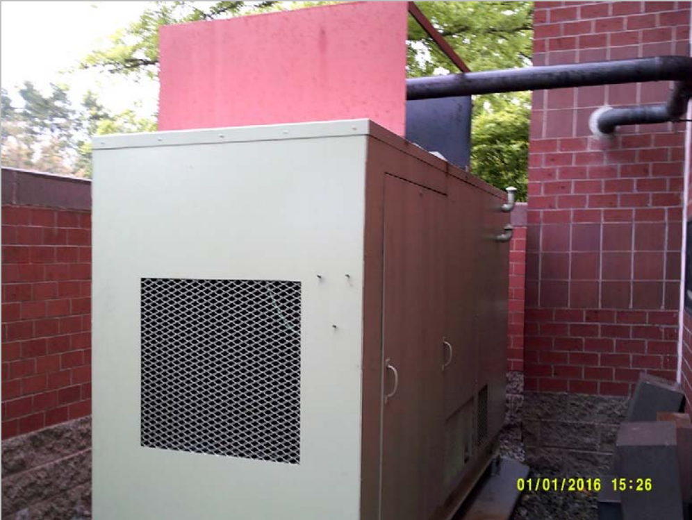
135Kw diesel generator for property
