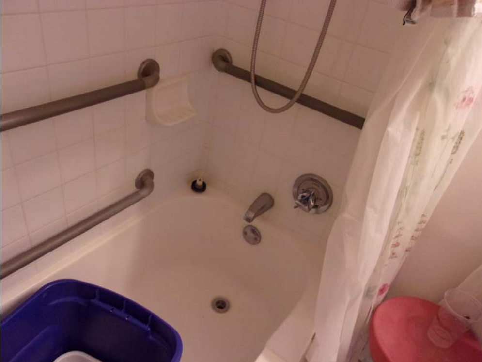
Handicap dwelling unit shower with grab bars, 60" shower hose, and levered hardware
