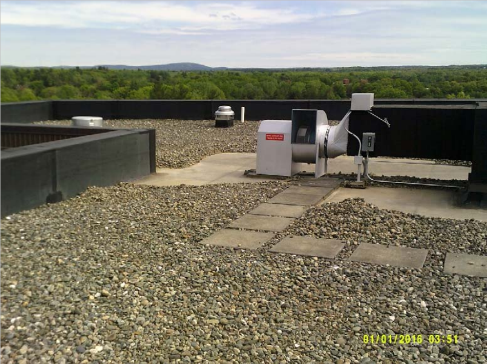
Coleman House II roof
