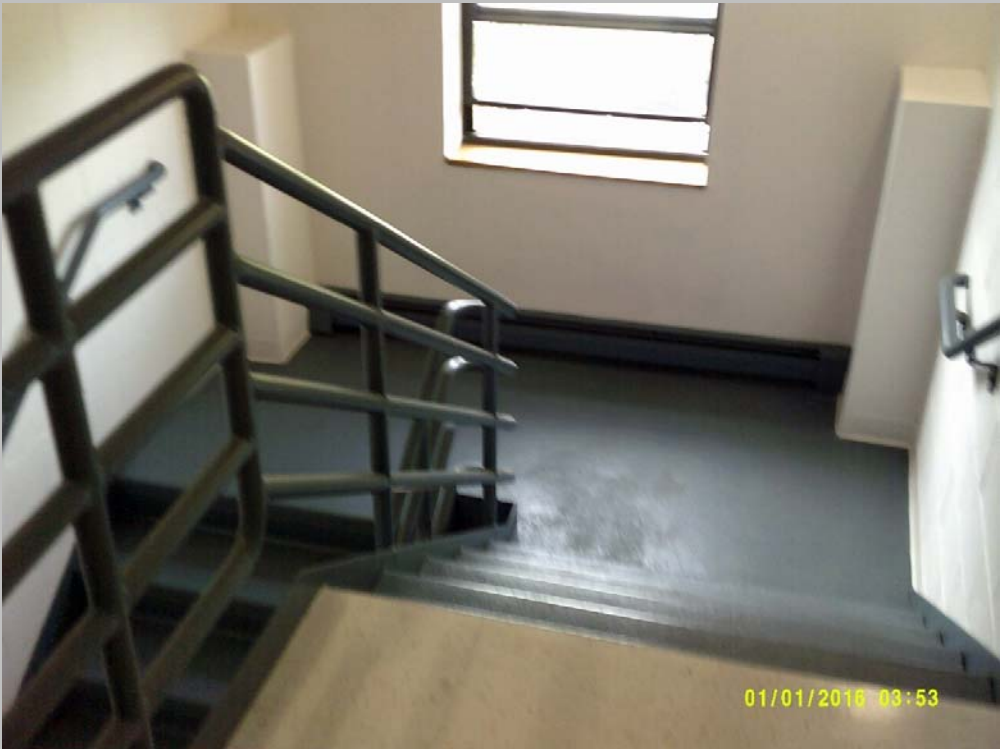
Property interior stairwell
