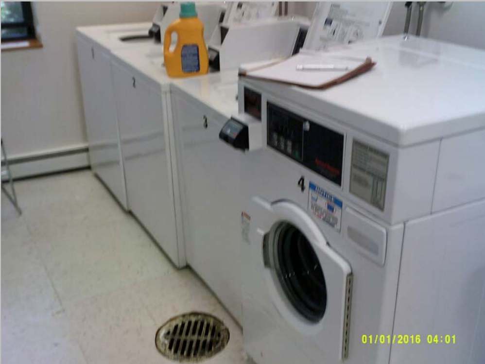
Common area laundry room
