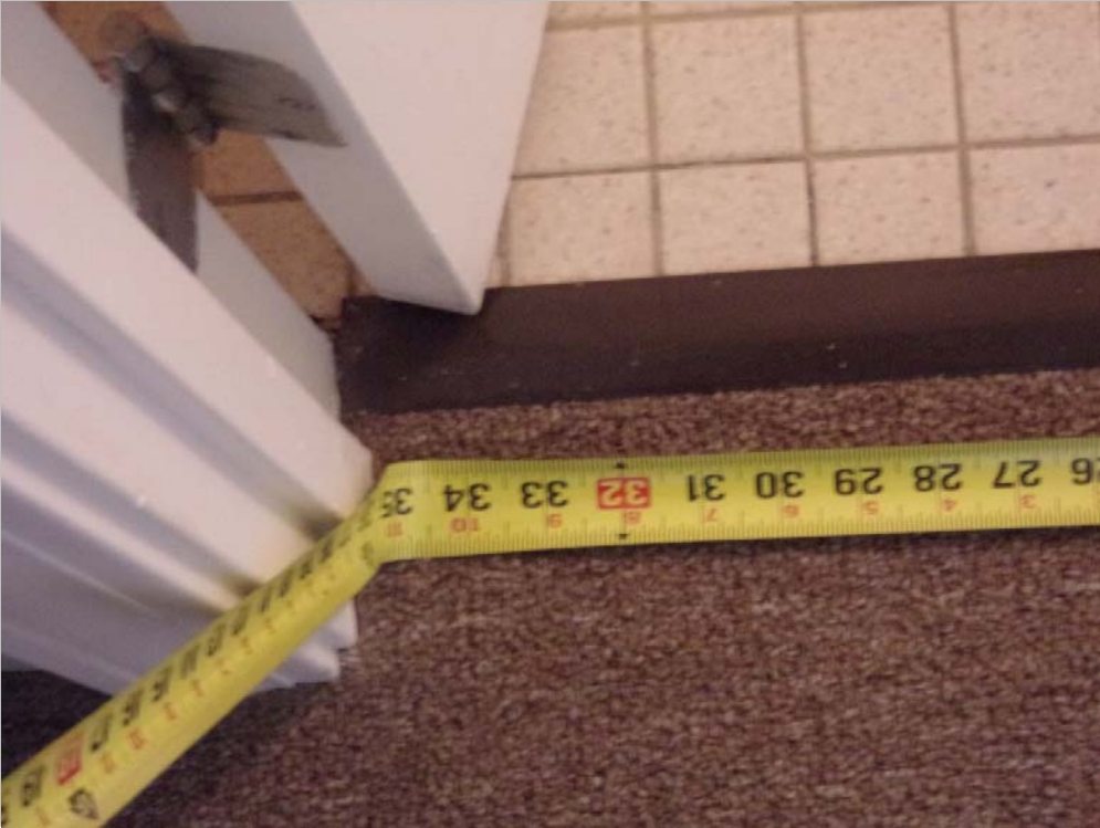
Handicap dwelling unit bathroom door opening width
