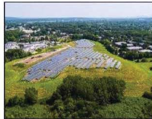
Renewable Energy: Solar array at Rumford Avenue
