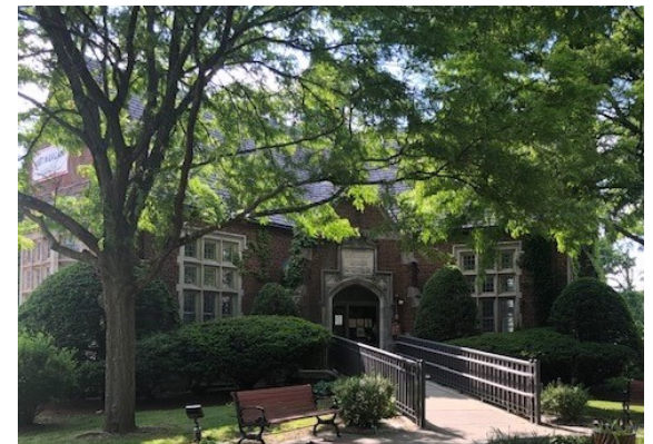
Photo of exterior entrance ramp at the Auburndale library
