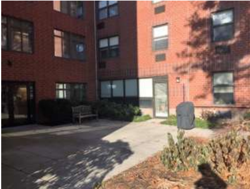
Front view of building exterior
