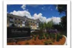
Shillman House Framingham, MA
