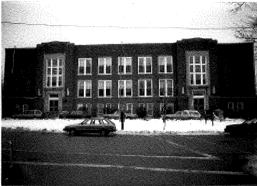
Davis School, 492 Waltham St (NWT.3884)
