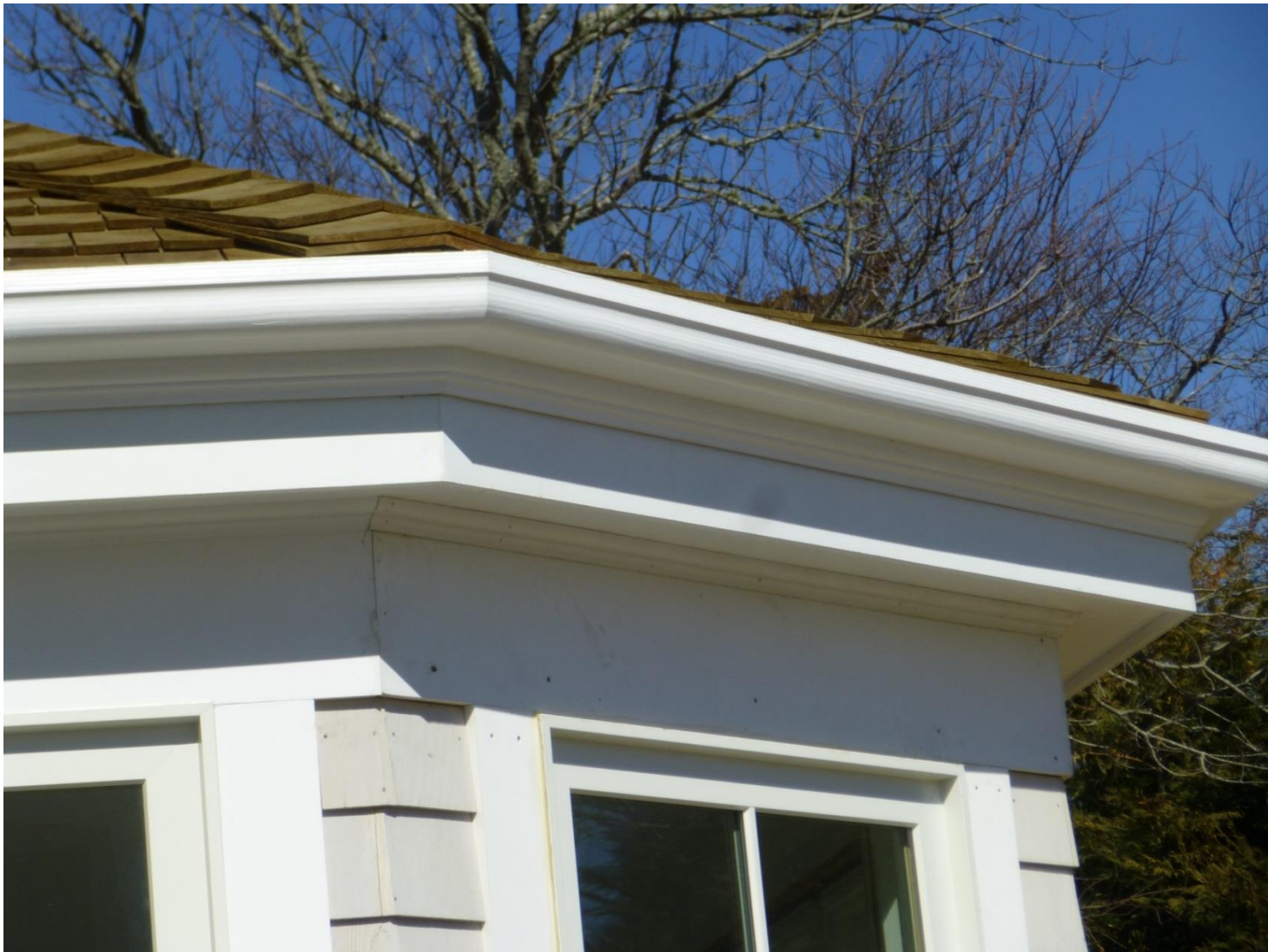
Old Harbor Lane - Chatham, MA
