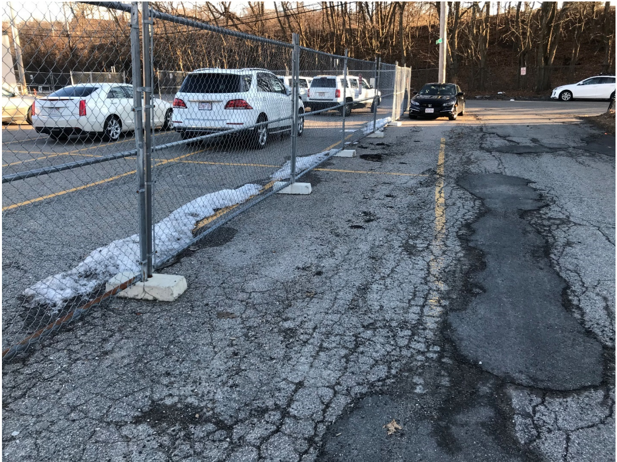
Parking stalls appear to be encroaching Harvey Place
