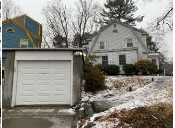
16 Crehore Dr garage to be demolished
