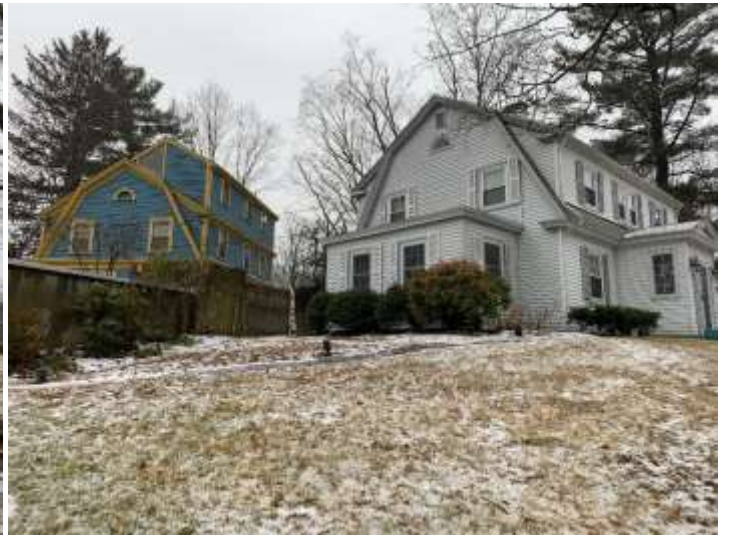
Small side addition to be replaced by garage and bedroom above
