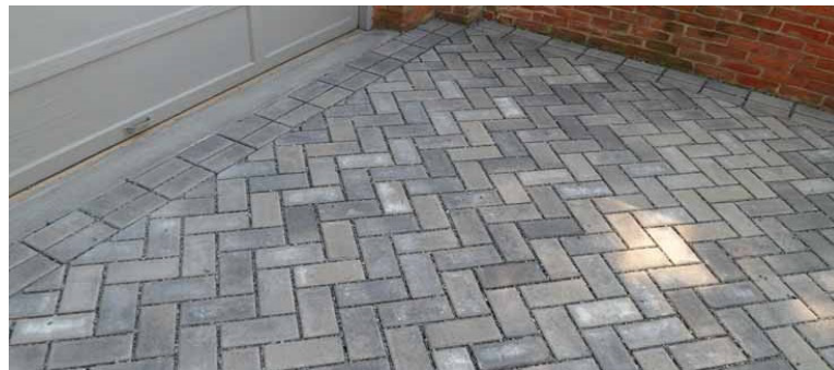
Permeable Driveway Pavers
