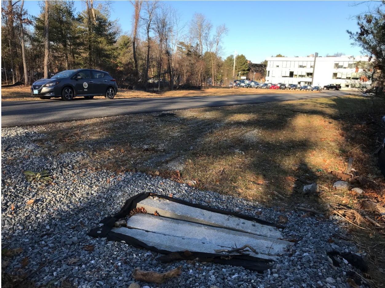
Some sort of drainage structure yet uncompleted.
