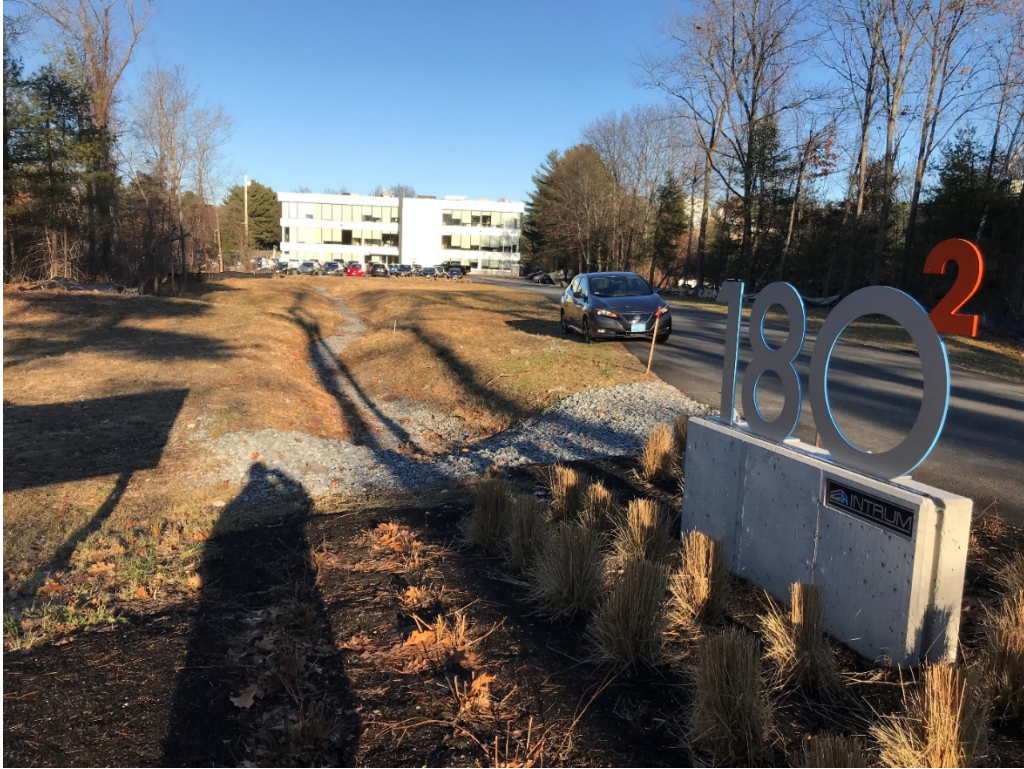
Drainage swale and new driveway apron
