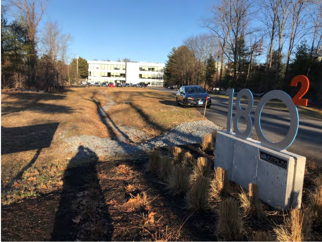
Drainage swale and new driveway apron
