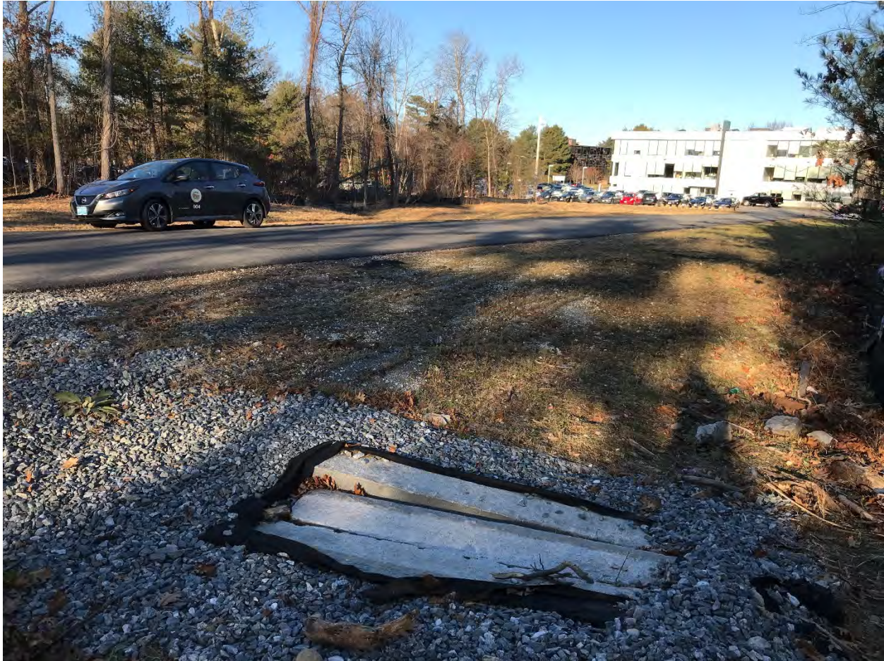
Some sort of drainage structure yet uncompleted.
