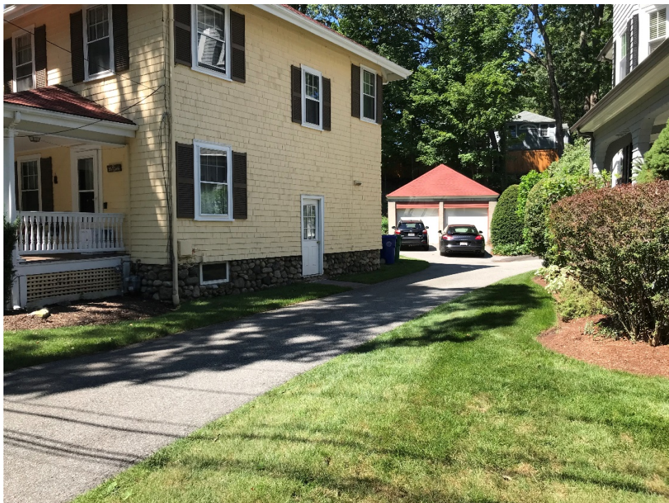
Looking towards the existing 2 stall garage
