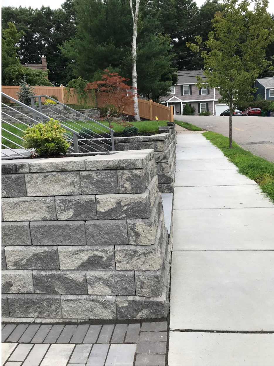
Retaining wall along Walsh Road looking towards Wiswall Road
