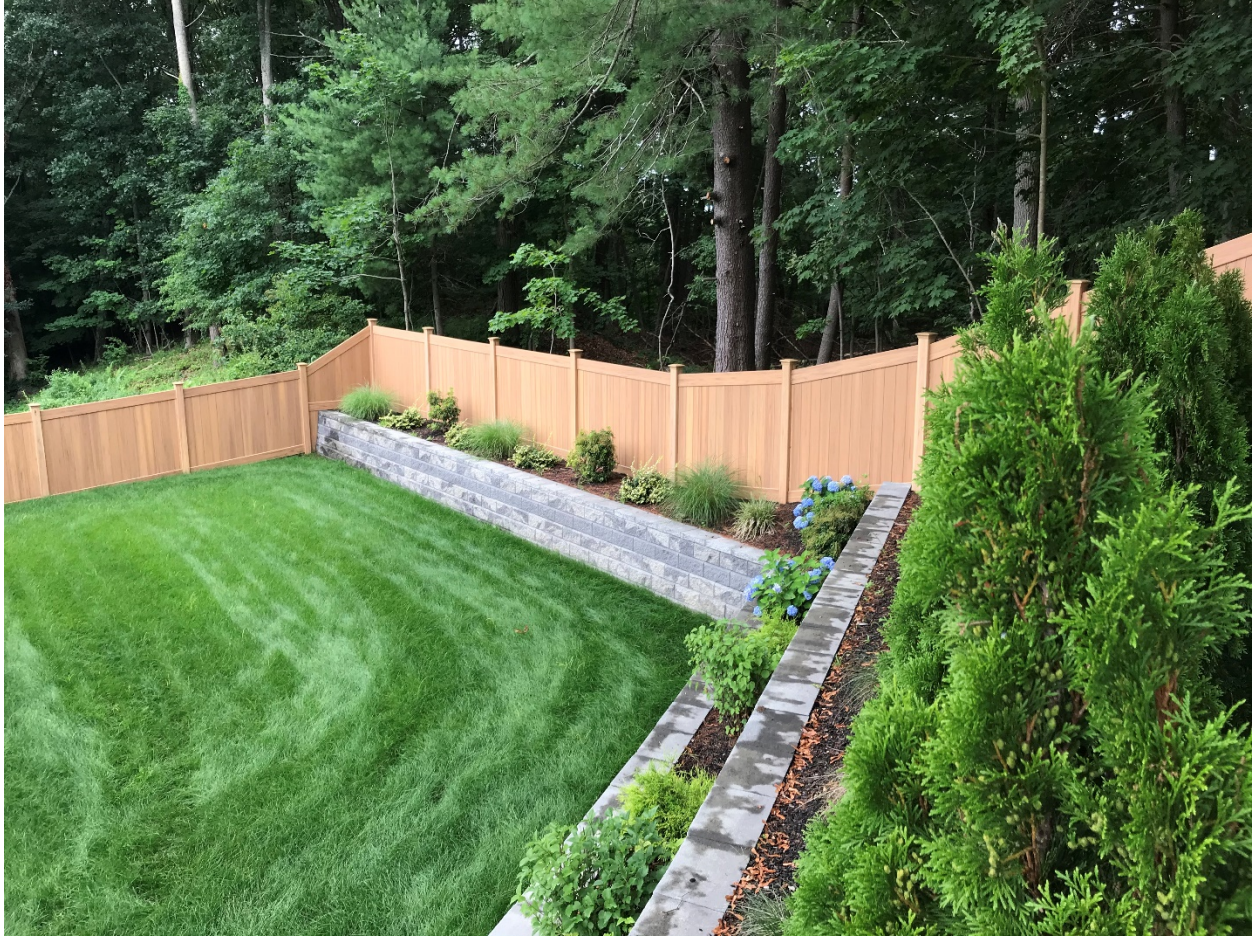
Retaining wall along Wiswall Road property line
