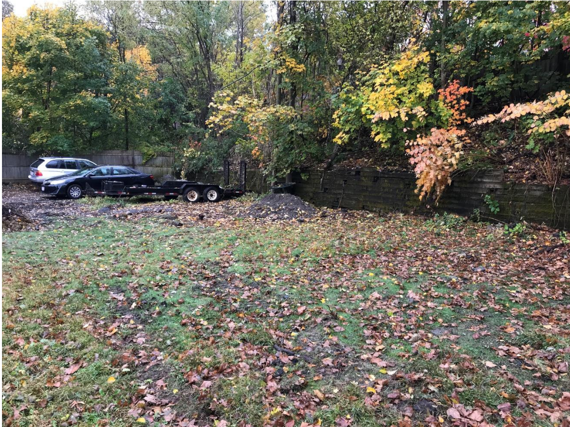
Existing wooden retaining wall along western property line
