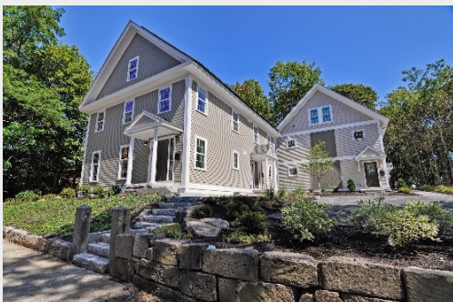
E+ Solutions Highland St. Project
