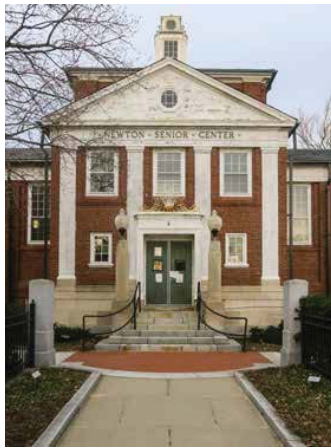
The outside stairs take you up three feet to a landing
