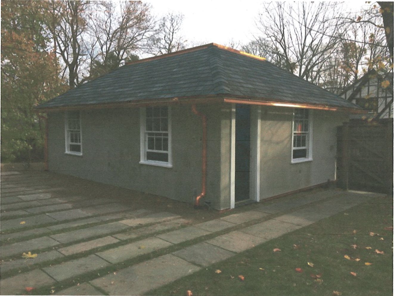
Alternate view, finished garage project
