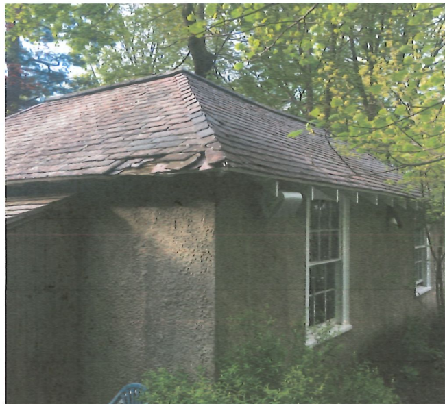
(1) ROOF: Remove, re-frame, and replace the roof.
