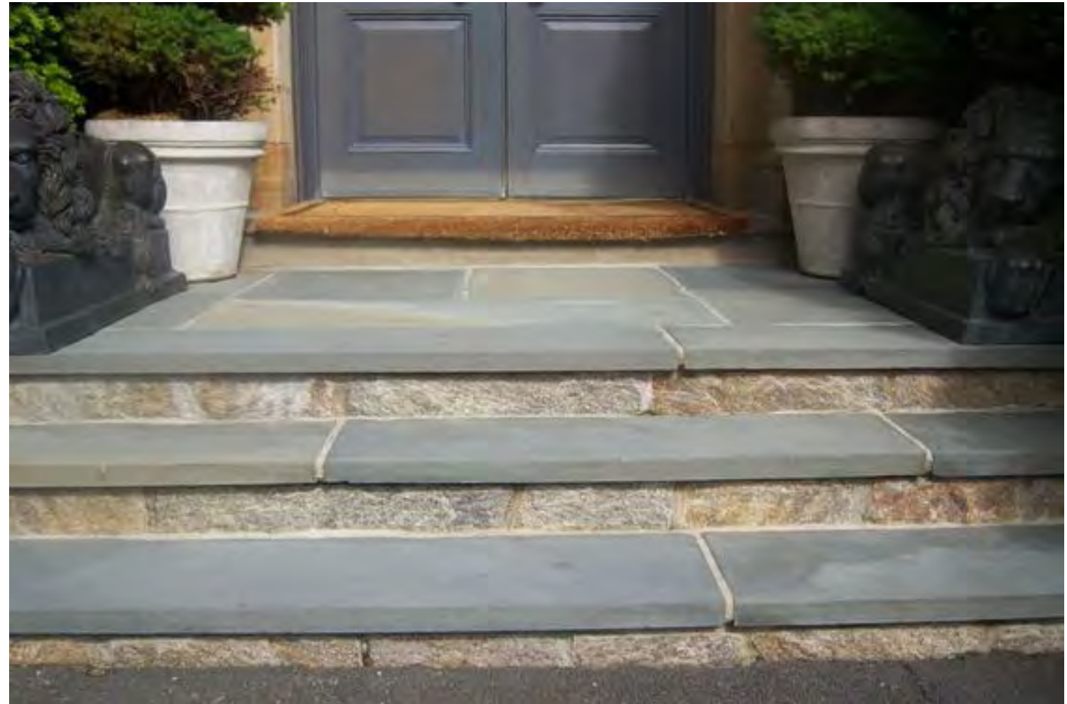
Example of Blue Stone Steps for Look we are Trying to Achieve
