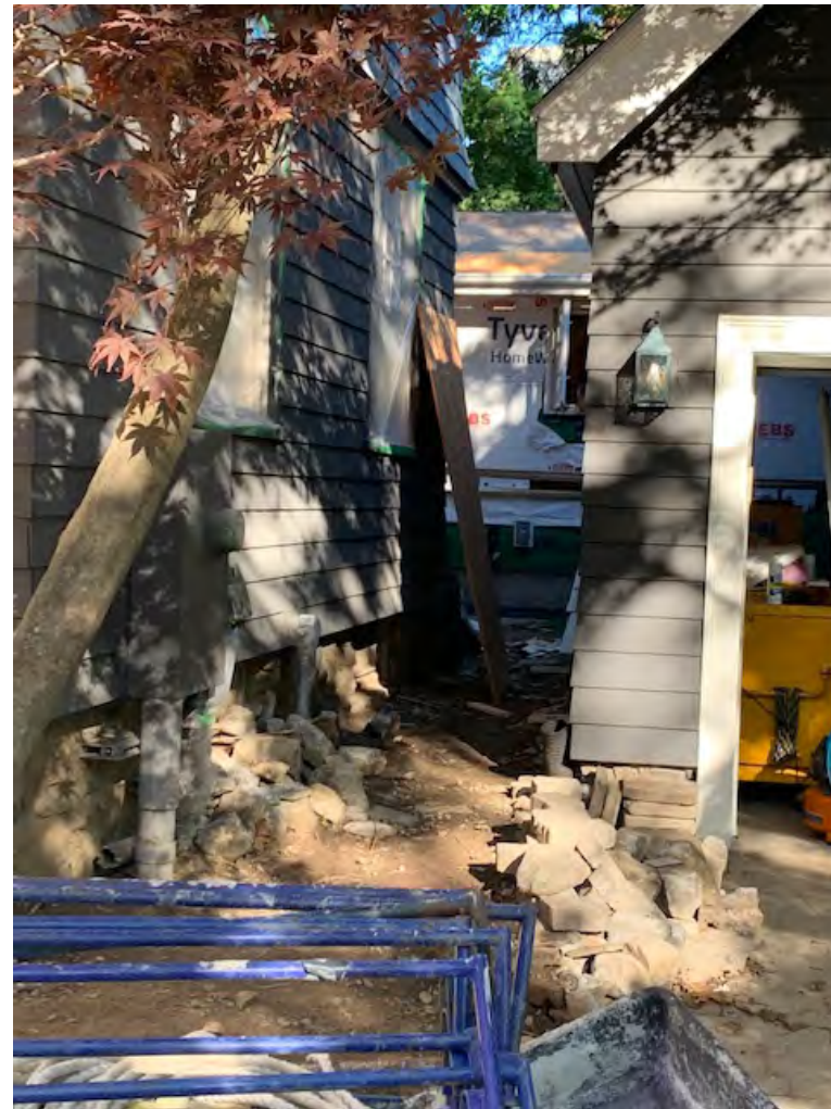
Close up of House/Garage Alley Proposed Gate Location
