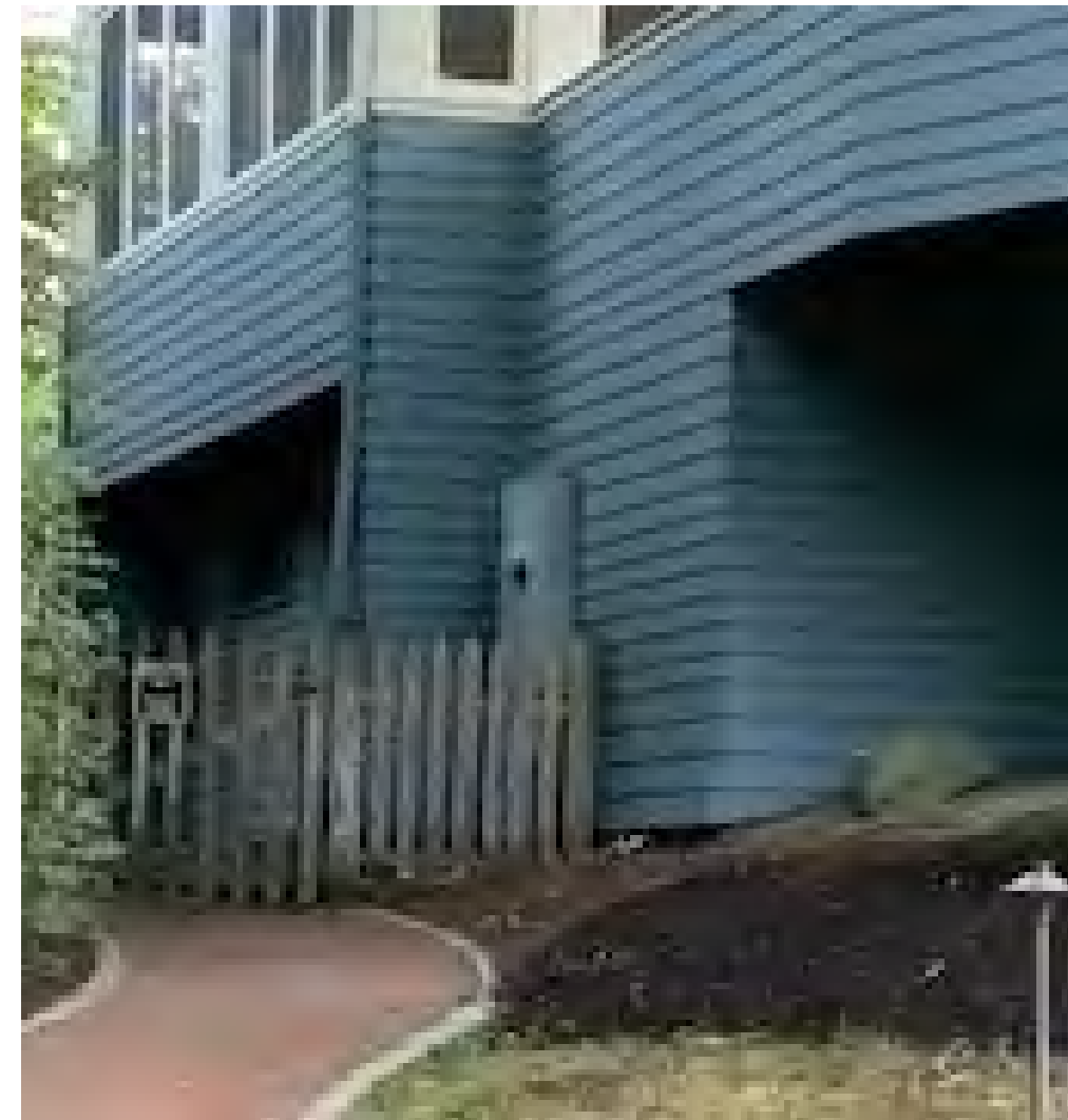
Enlarged View: Similar Electrical Box at 121 Suffolk Road
