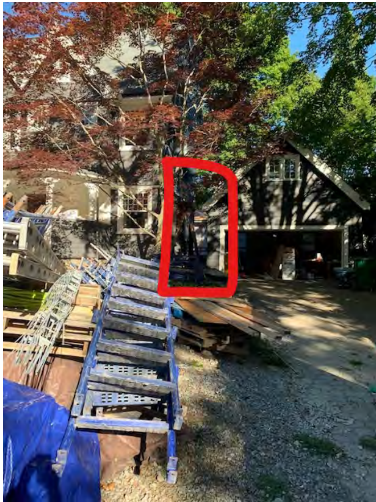
View of House/Garage Alley from Street
