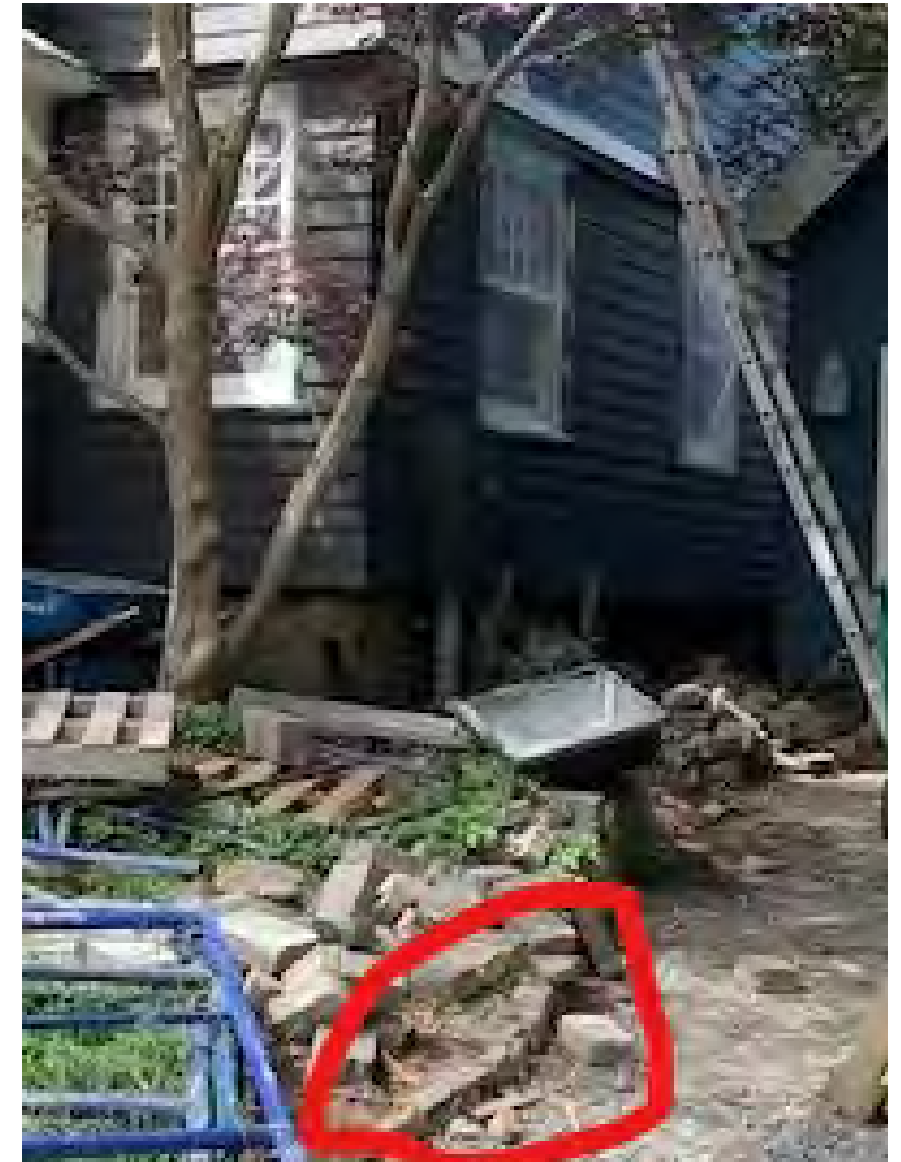
Existing Curbing to be Reused
