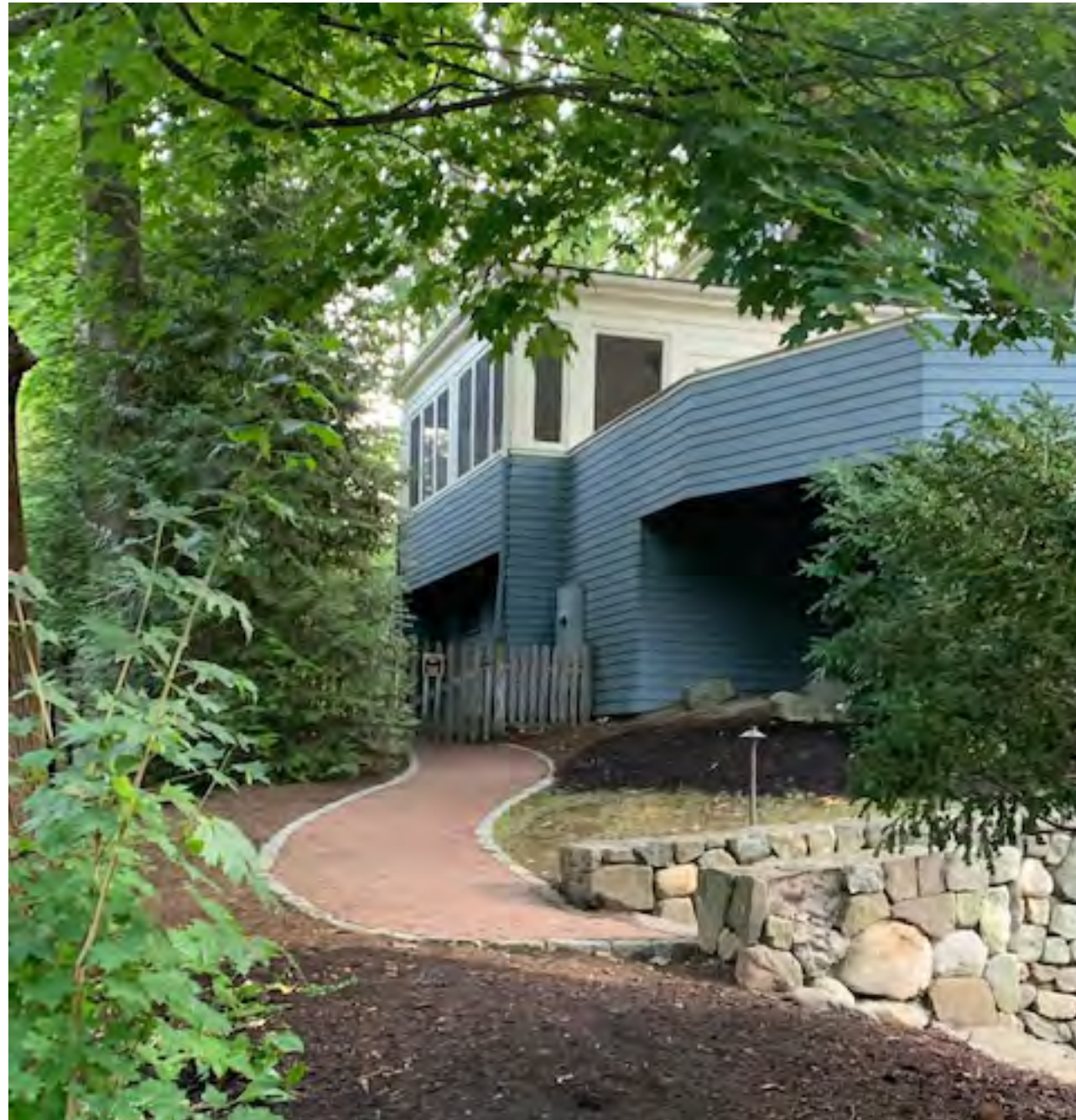
Similar Electrical Box at 121 Suffolk Road (View from Street)
