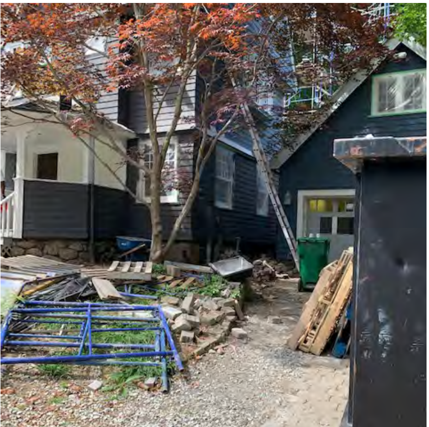
New Electrical Box (Same Location) Painted
