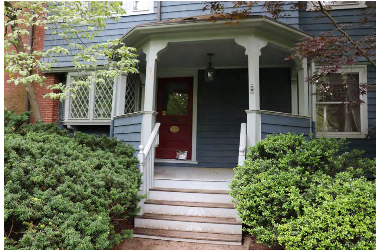
EXISTING FIXTURE - DANGEROUSLY LOW
