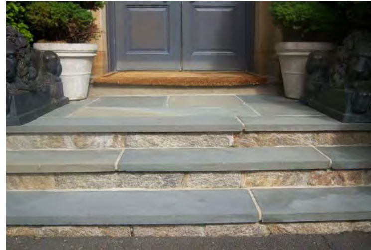
Example of Blue Stone Steps for Look we are Trying to Achieve
