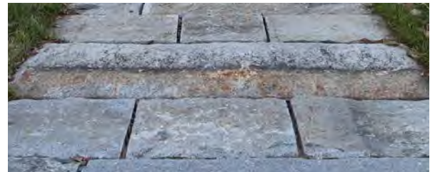
Reclaimed granite curb pieces, for edging and steps.
