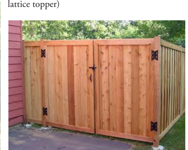
Double gate at new fence
