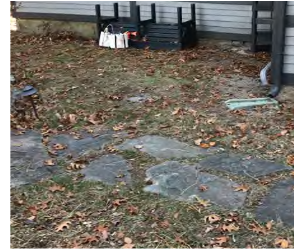
Wide-set flagstone pavers with lawn joints. Use existing material for inspiration.
