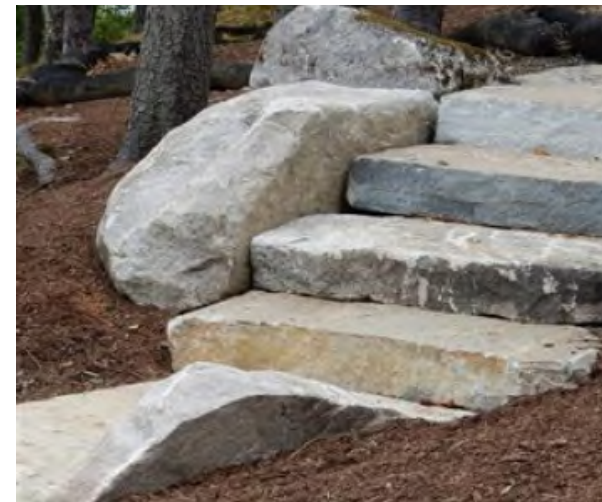
Boulders flanking stairs, set among paving and planting.
