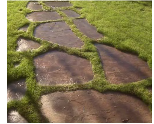
Wide-set flagstone pavers with lawn joints. Use existing material for inspiration.
