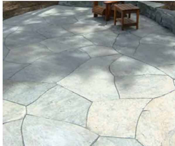
Mosaic style cut flagstone - tight jointing. Use existing flagstone as inspiration for new material.
