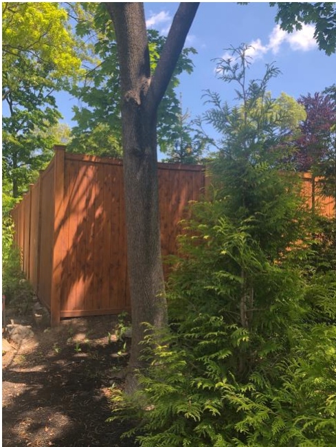
Fence transition from 8 ft. to 6 ft.:
