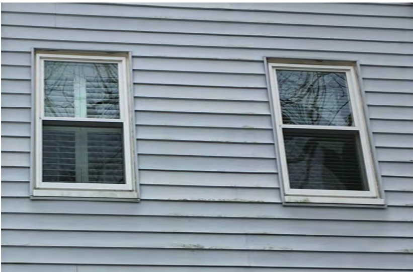
REST OF HOUSE WINDOW TRIM
