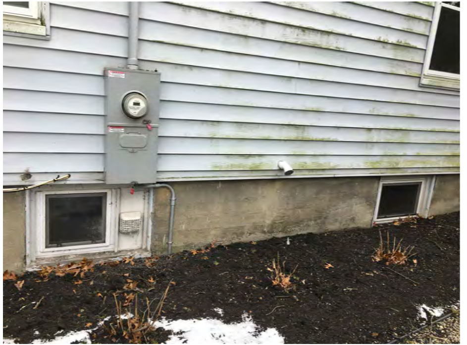
EXISTING EXPOSED CONCRETE FOUNDATION
