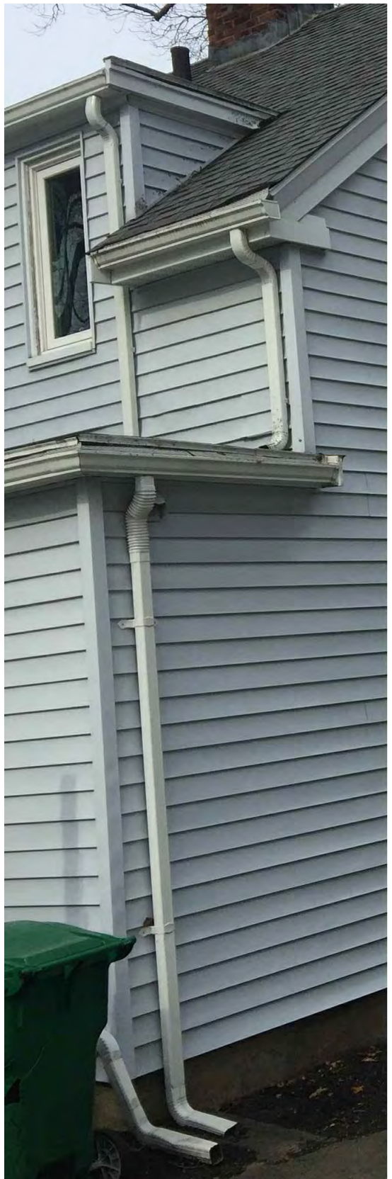
EXISTING GUTTERS & DOWNSPOUTS
