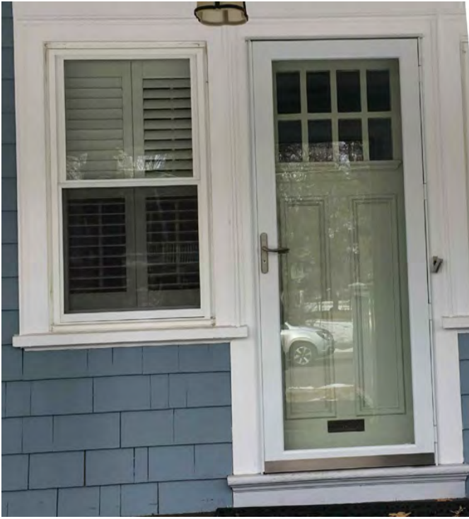
FRONT PORCH DOOR/WINDOW TRIM
