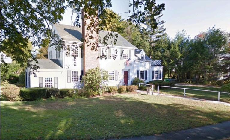
EXISTING HOUSE PRE-RENOVATION & ADDITIONS
