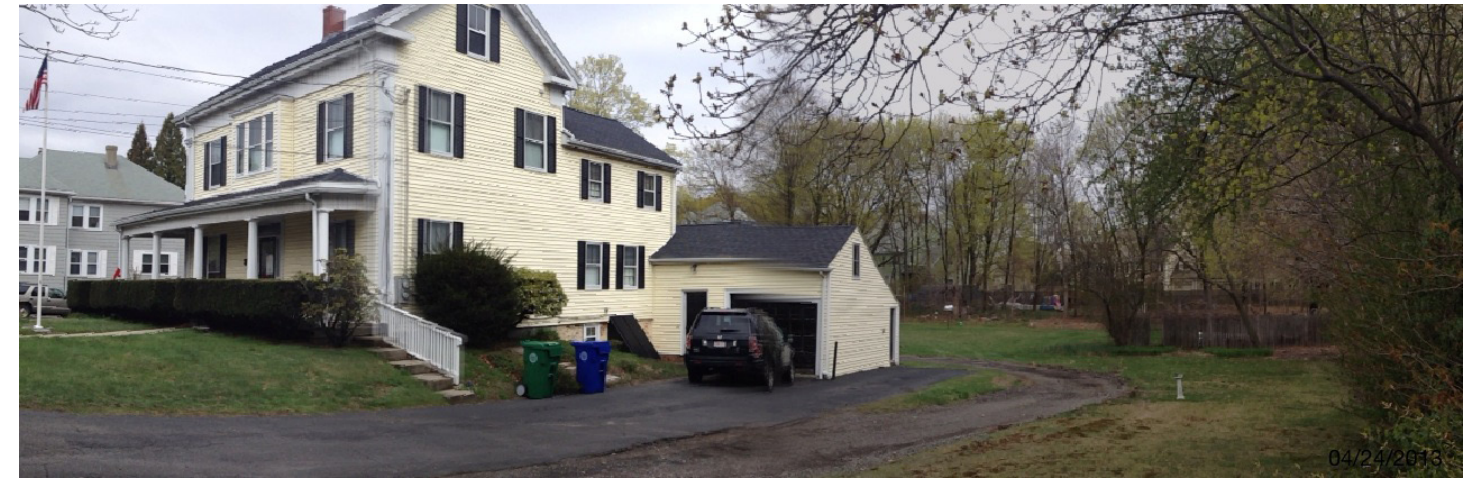
VIEW FROM AUBURN ST
