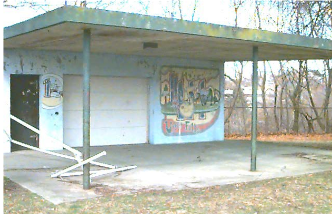
Storage Structure in Upper Falls Playground
